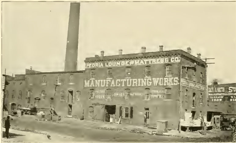
OFFICE OF STUBER & KUCK, 201-203 N. WATER ST.
