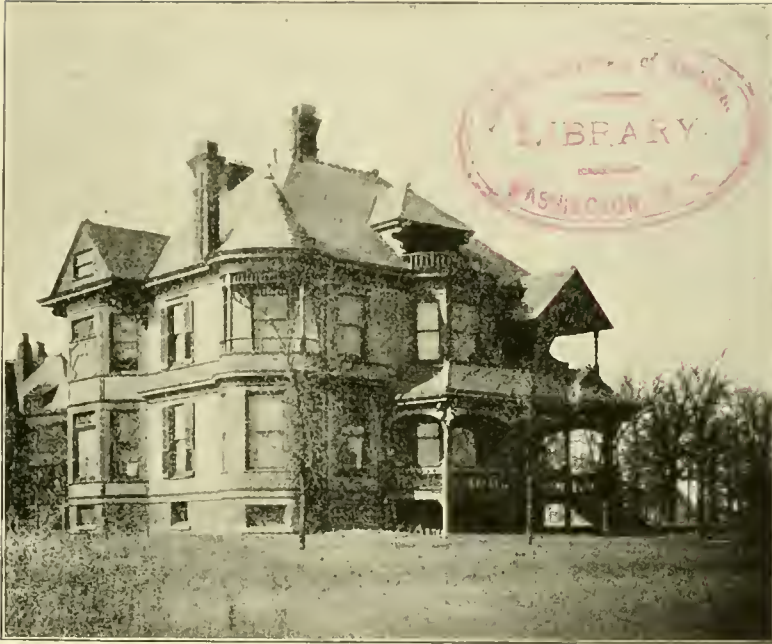
RESIDENCE OF JUDSON STARL, 211 CRESCENT AVE.
