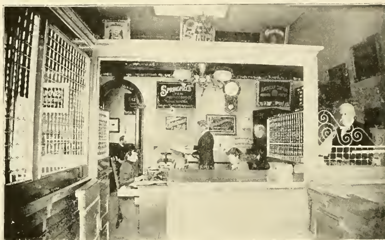
OFFICE OF C. M. BROWN, 214 MAIN ST.
