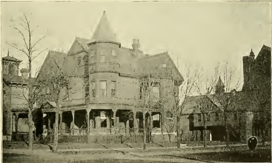
RESIDENCE OF H. H. FAHNESTOCK, 200 PERRY STREET.
