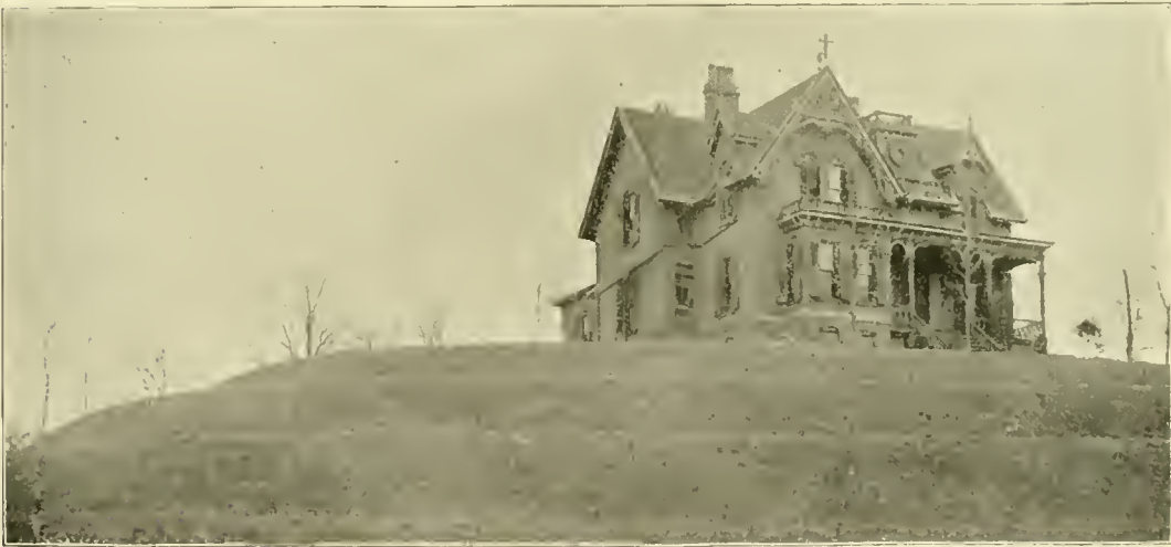
RESIDENCE OF T. A. TURNER, 1303 BLUFF STREET.
