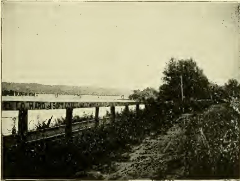
ROAD FROM NARROWS SHOWING FREE BRIDGE.
