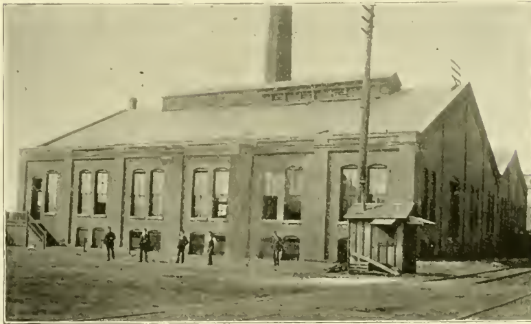
JENNEY ELECTRIC LIGHT AND POWER CO., WATER, COR. LIBERTY ST.
