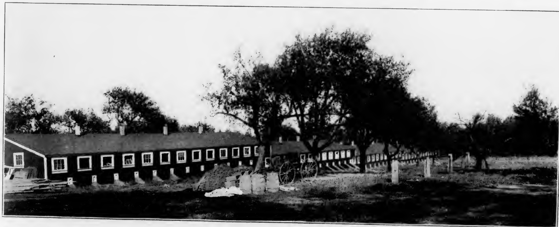
A Brooder House, 20 x 250 feet. Double pipe brooder system. 200 hovers. Capacity 10,000 chicks. This brooder house is one of the buildings at Pittsfield Farm, Box 265, Pittsfield, Me., where a lot of Barred Rock aristocracy has its birth.
