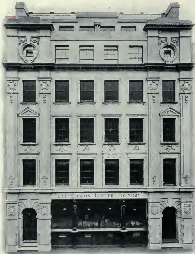
OFFICES & WAREHOUSES : 82 & 83 CHISWELL ST., LONDON, E.C.
