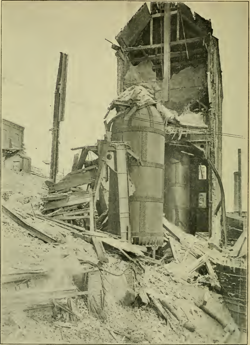
FIG. 2. VIEW LOOKING INTO THE WRECKED DIGESTER HOUSE.
