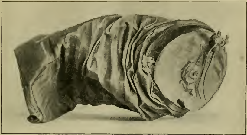
AN EXPLODED PEANUT ROASTING BOILER.
