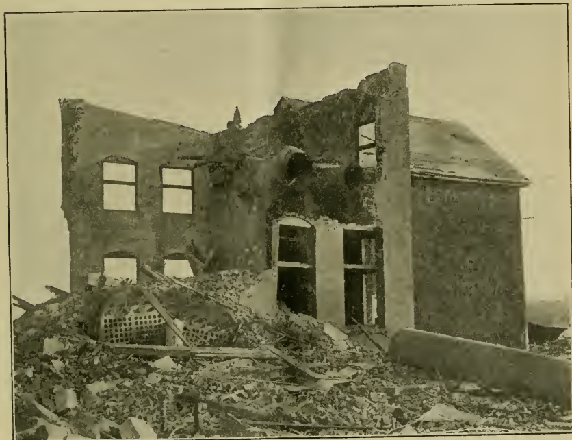
FIG. 4. WRECKED BOILER HOUSE.
