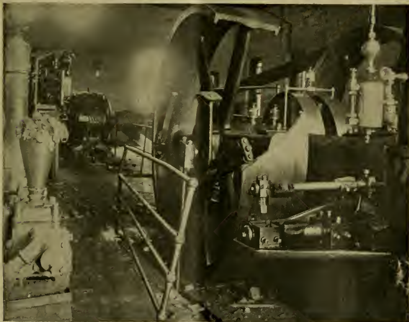
FIG. 1.— SHOWING THE BROKEN WHEEL AND GOVERNOR.
