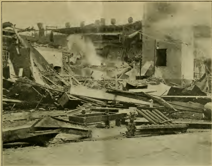
FIG. 4. SHOWING PORTIONS OF THE NO. 2 ECONOMIZER STANDING ON ITS PLATFORM JUST BACK OF THE STACK.
