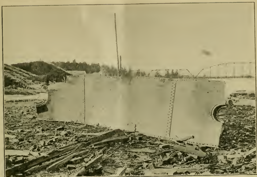
FIG. 3. RUPTURED MANHOLE COURSE "B."
