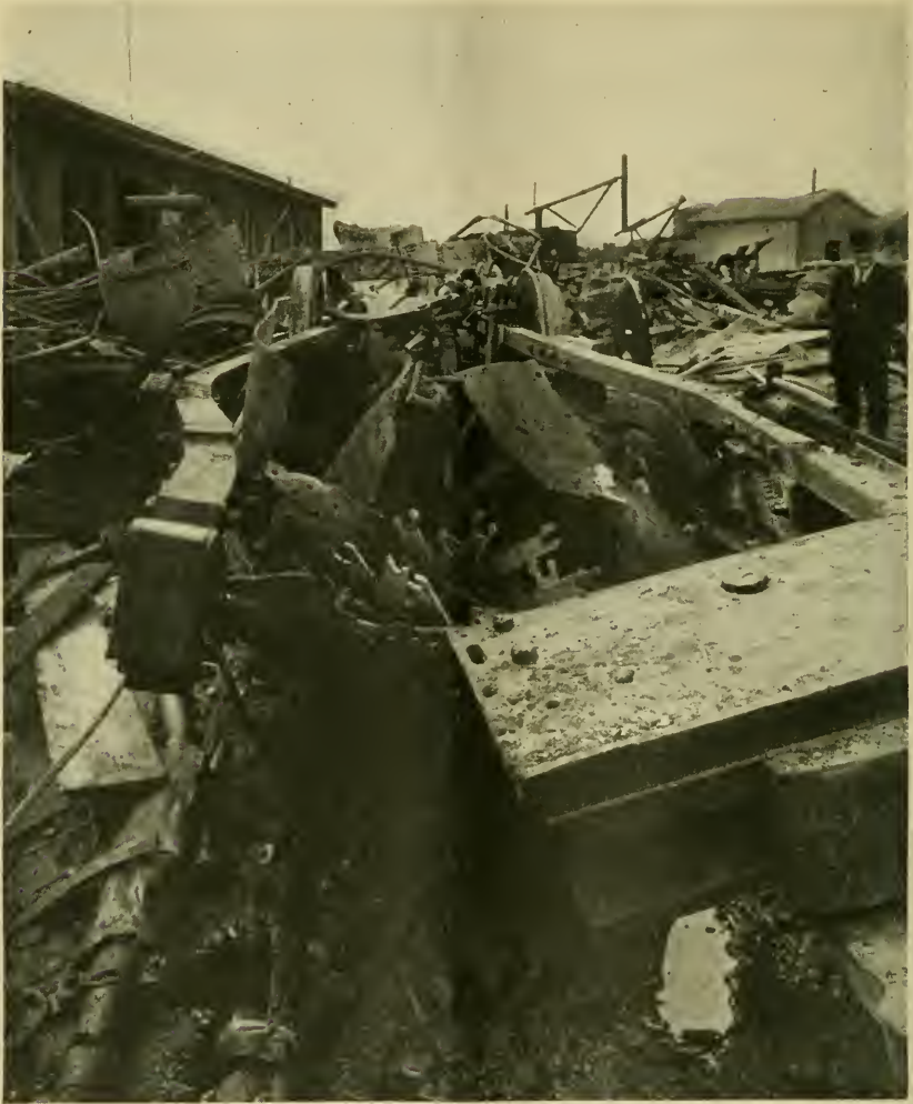
FIG. 1. SHOWING BROKEN SLING STAYS.
