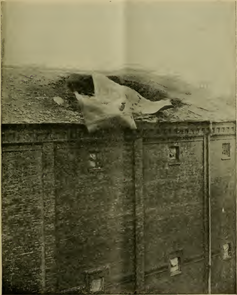
FIG. 3.—RUPTURED STEAM DRUM ON THE REFRIGERATOR HOUSE ROOF.
