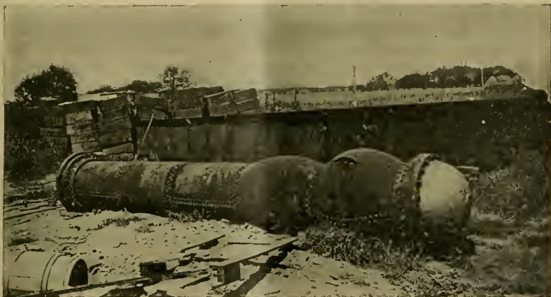
ILLUSTRATING THE STIFFNESS OF A GIRTH JOINT.
