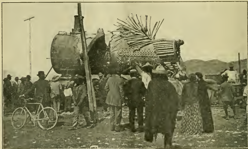
BOILER EXPLOSION AT SALTILLO, MEXICO. No. 270 IN JUNE LIST.
