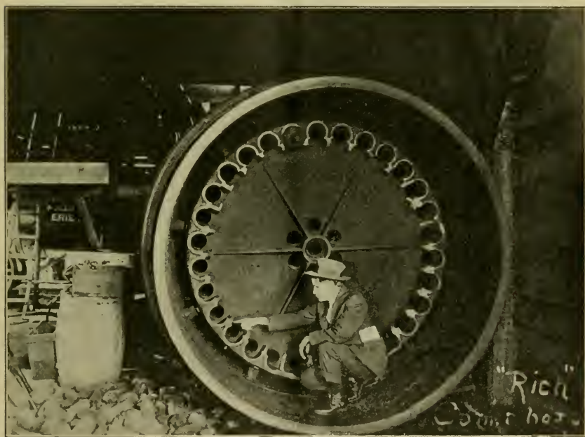
FIG. 3.—THE INSIDE OF THE EXPLODED DRYER HEAD. THE MAN IS POINTING TO ONE OF THE OLD BREAKS.
