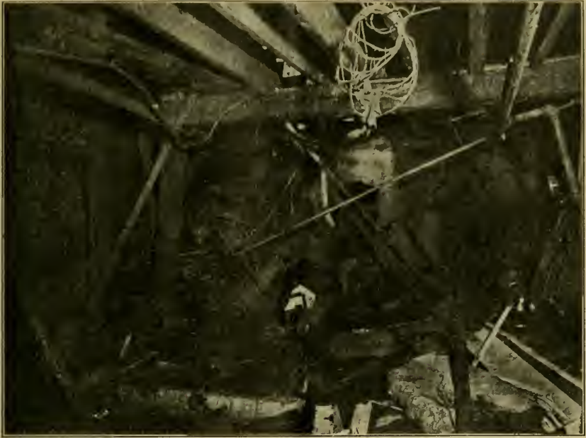
FIG. 1.—THE WRECKED BOILER ROOM, SALEM BANK AND TRUST COMPANY, SALEM, ORE.
