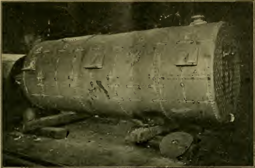
FIG. 4. BOILER 4092 PRIOR TO THE TEST. NOTE THE 10-INCH GAGED LENGTHS.
