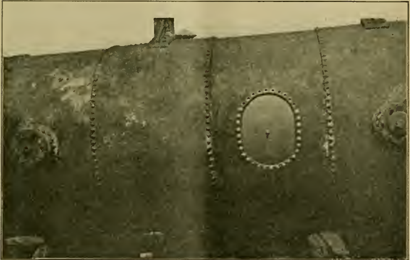
FIG. 3. APPEARANCE OF BOILER 303 AFTER TESTING.
