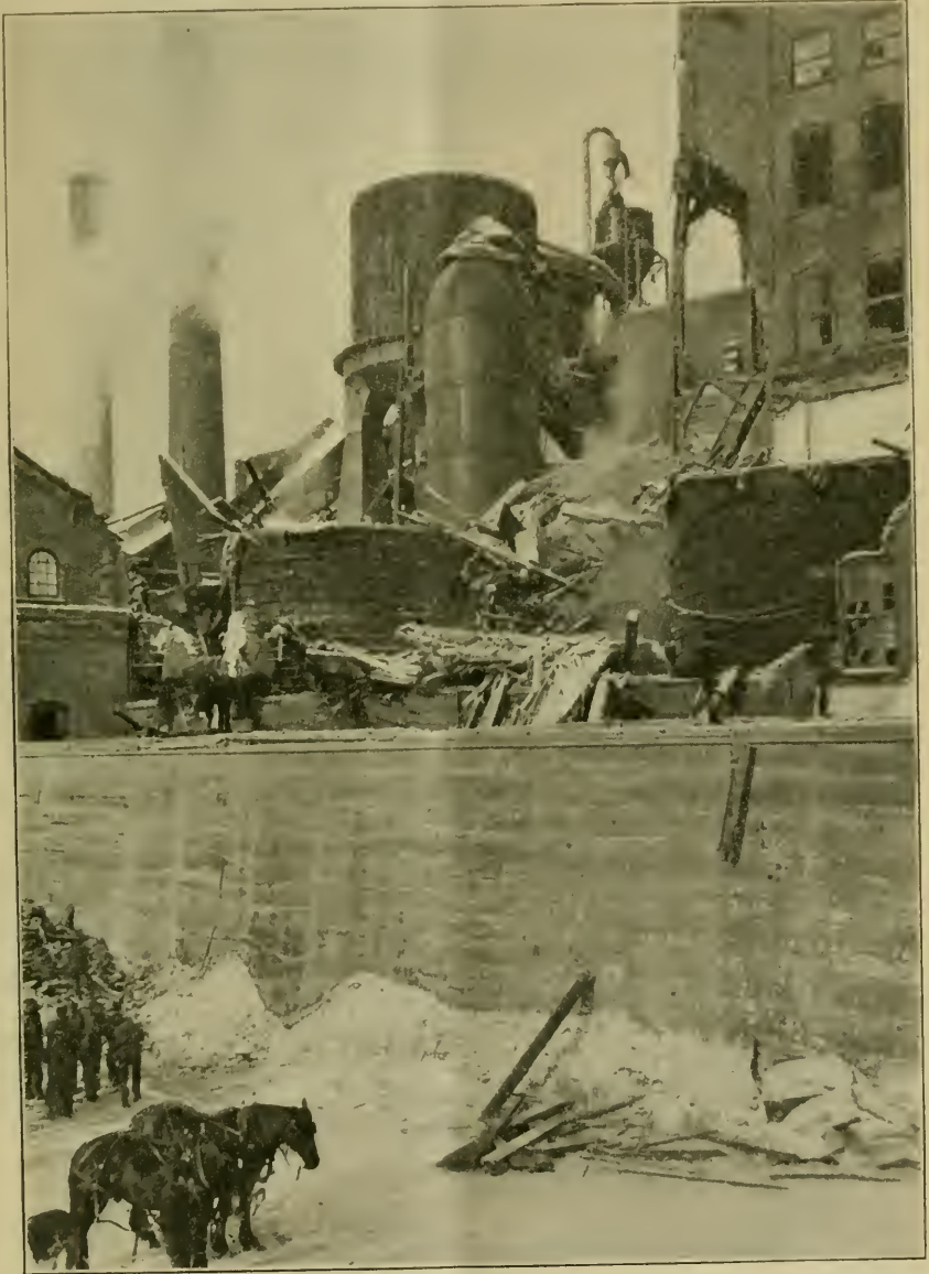
FIG. 1. GENERAL VIEW OF THE DESTRUCTION AT GRAND MERE.
