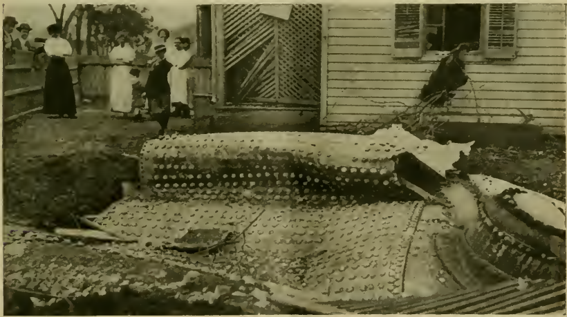
FIG. 2. WRAPPER SHEET AND DOME IN DOOR YARD.
