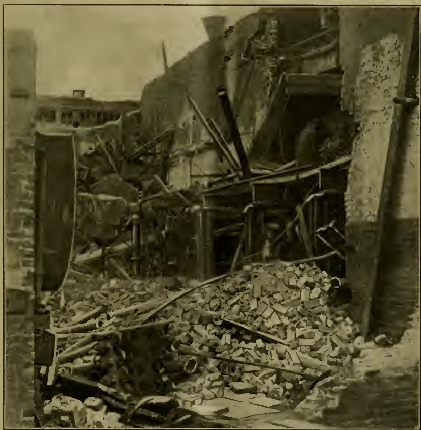
FIG. 5. A NEAR VIEW OF THE WRECK. ECONOMIZER EXPLOSION AT SAYLESVILLE, R. I.
