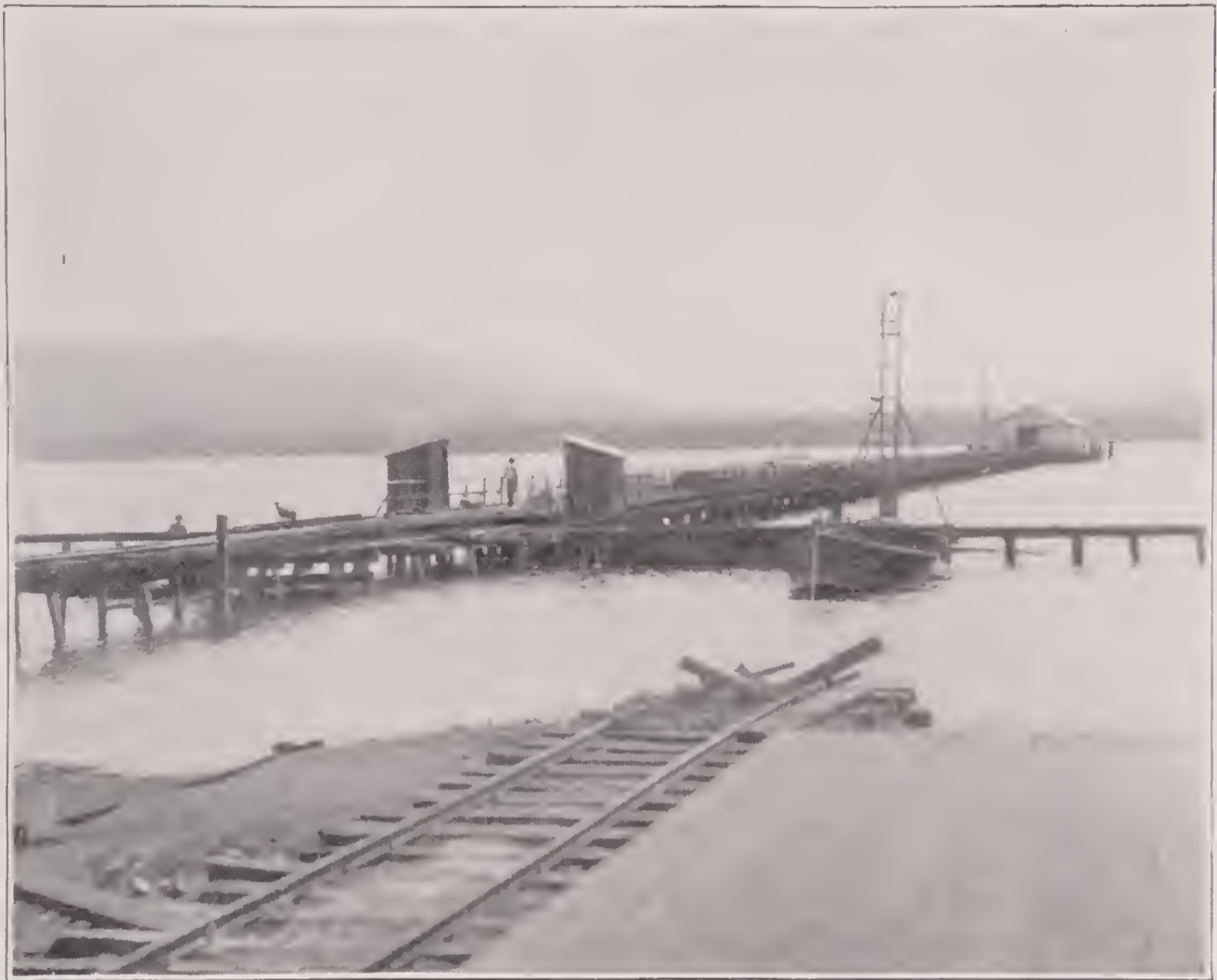
Pier at Puerto Barrios.
