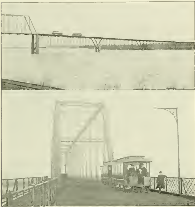
THE MISSOURI RIVER BRIDGE.
