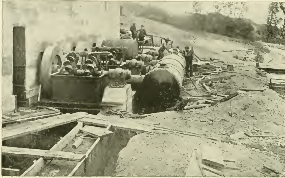
FIG. 4—ARRANGEMENT OF FLY-WHEELS, RECEIVERS AND BUCKETS.
