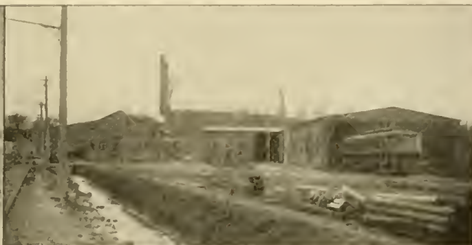
POWER HOUSE AND CAR BARN.
