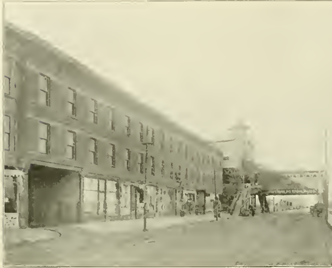
FIG. 1—CALUMET TERMINAL STATION.
