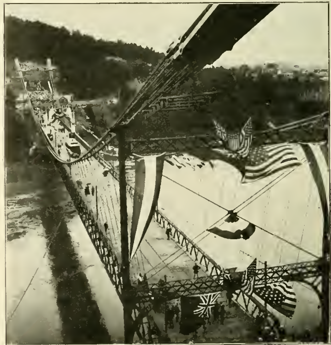
FIG. 3—LEWISTON BRIDGE OPENING DAY.
