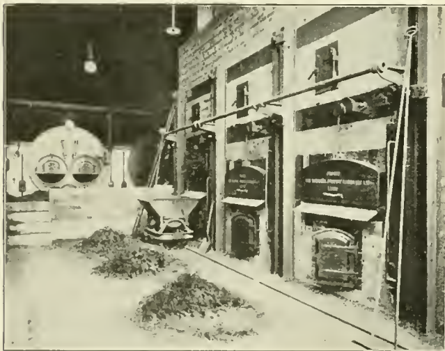
FIG. 4- DESTRUCTOR AND PART OF BOILER HOUSE.
