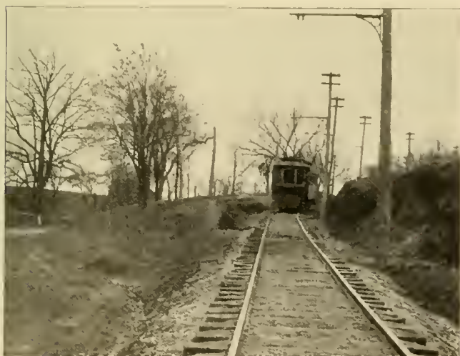
TRACK AND LINE WORK.
