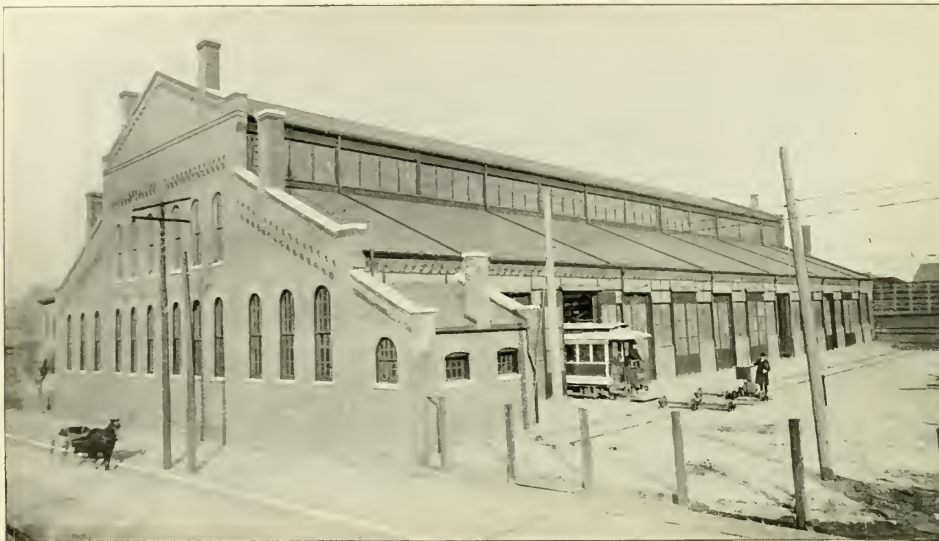
REPAIR SHOP OF LOUISVILLE RAILWAY CO.
