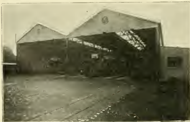
FIG. 11. END OF CAR SHED.
