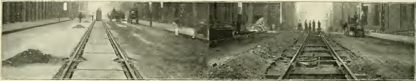
CONCRETE CONSTRUCTION IN PAVED AND UNPAVED STREETS.
