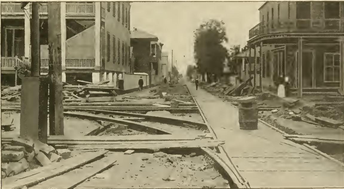
CULVERT CROSSING, ST. CHARLES STREET R. R., NEW ORLEANS.
