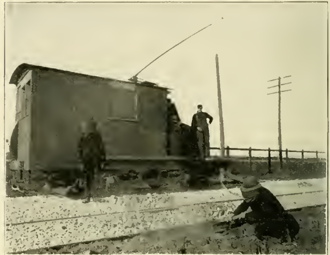
FIG. 7. CLEANING JOINTS.
