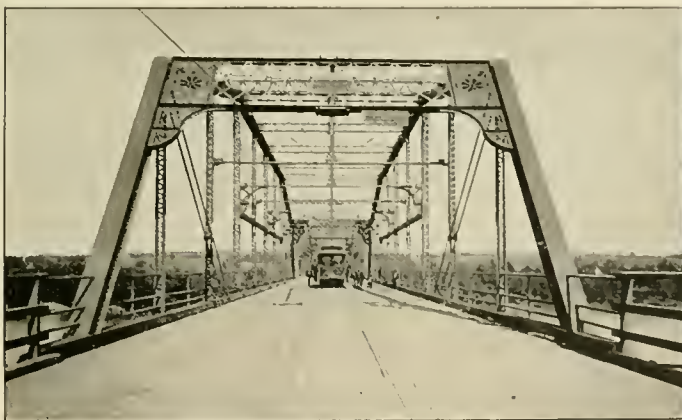
BRIDGE ON LINE OF NORTH AUGUSTA STREET RAILWAY.
