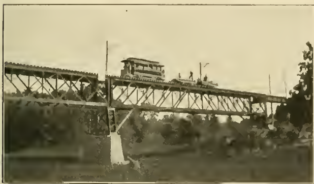
BRIDGE OVER PECK'S POND.
