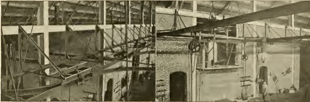
VIEWS OF TRAVELER SYSTEM IN SHOP.
