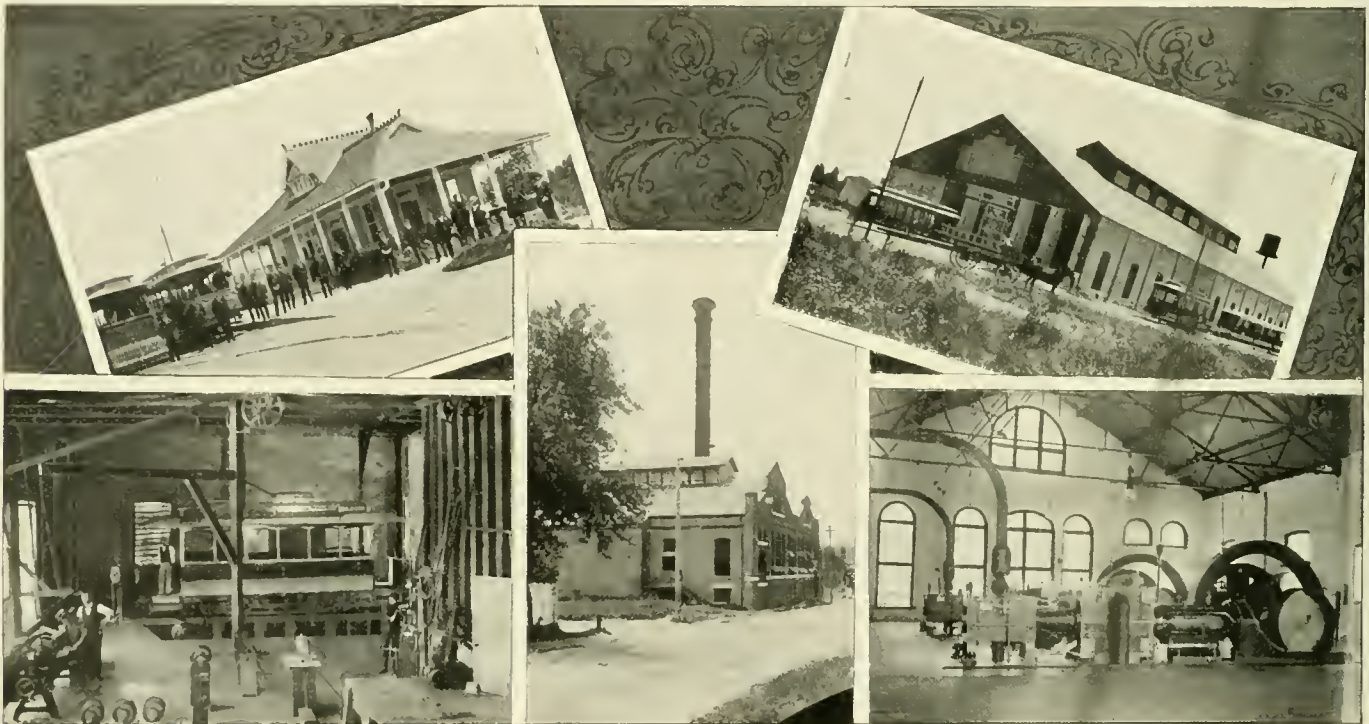
RESERVOIR PARK TERMINAL. REPAIR PIT.
