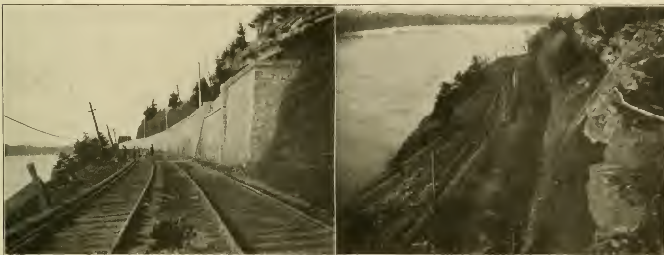
NEW YORK APPROACH TO NEW SUSPENSION BRIDGE AT LEWISTON, N. Y.
