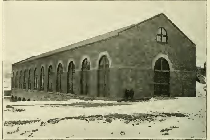
EXTERIOR OF POWER HOUSE.
