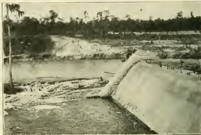
DAM AFTER THE EXPLOSION.
