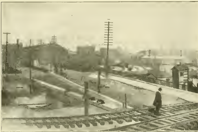
FIG. 2. VIEW OF VIADUCT.
