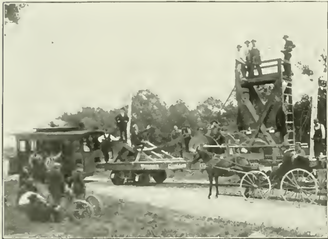
FIG. 3 STRINGING OVERHEAD WIRES.
