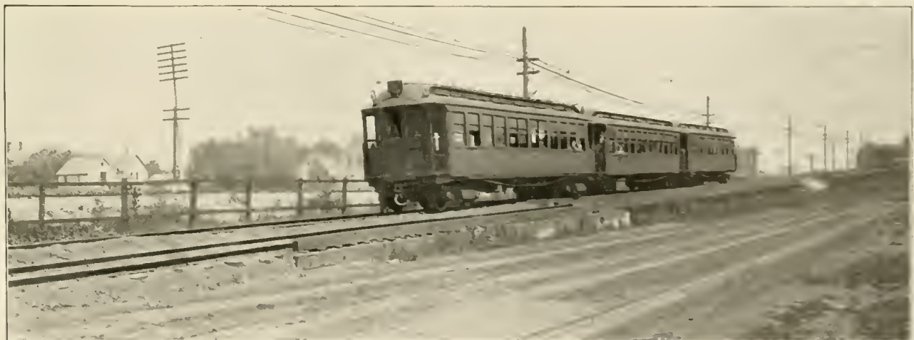
INCLINE OF LAKE STREET ELEVATED AT WEST 52D ST.
