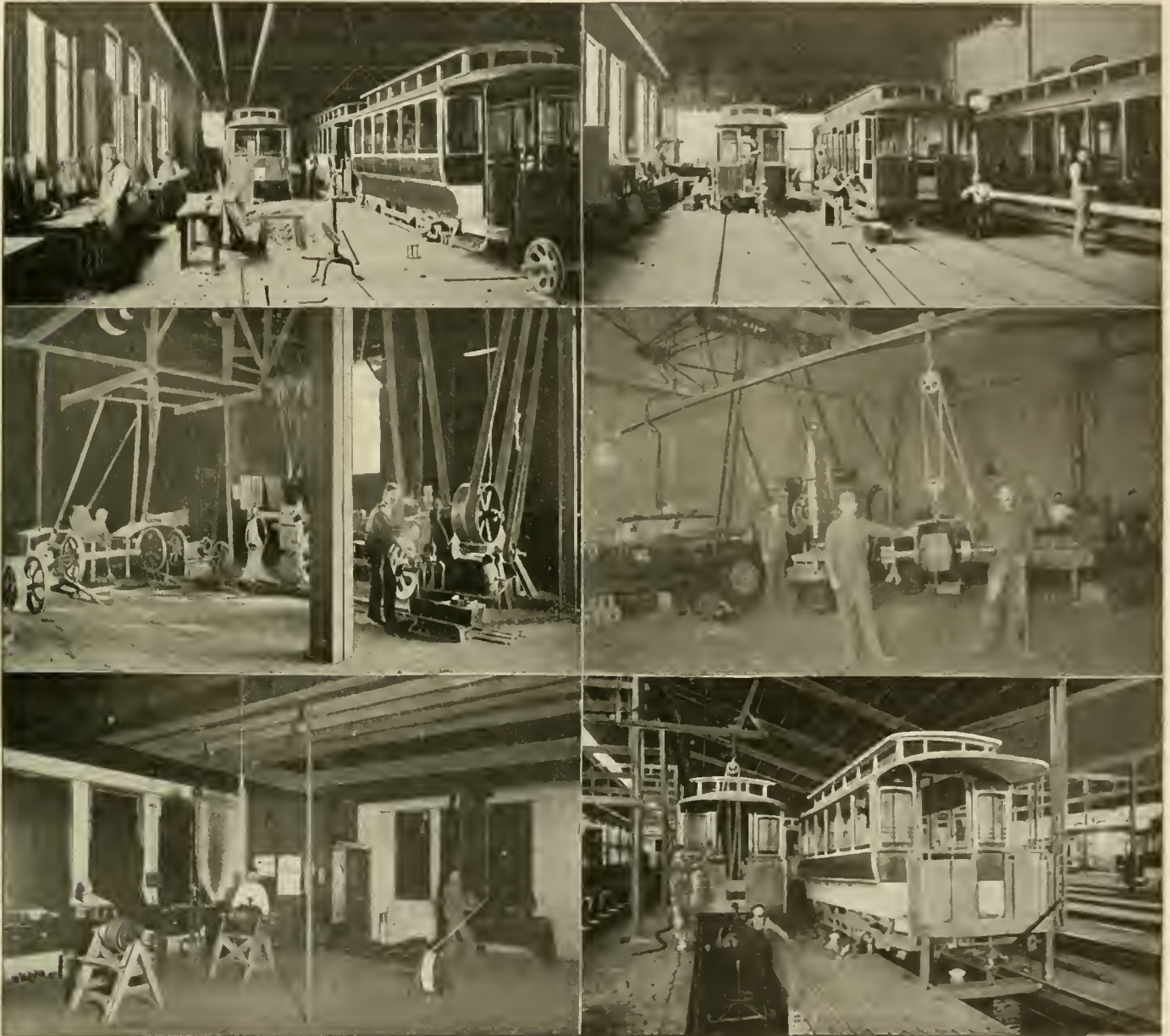
FIG. 3-CARPENTER SHOP. FIG. 5 MACHINE SHOP. FIG. 7-MOTOR WINDING ROOM.
