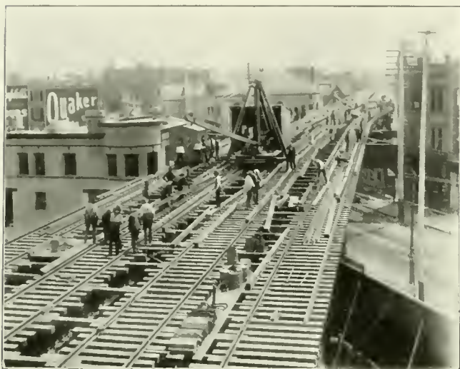
WORK ON THE NORTHWESTERN ELEVATED.
