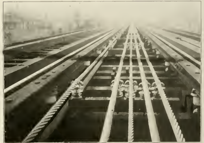
FEEDERS, SOUTH SIDE ELEVATED, CHICAGO.
