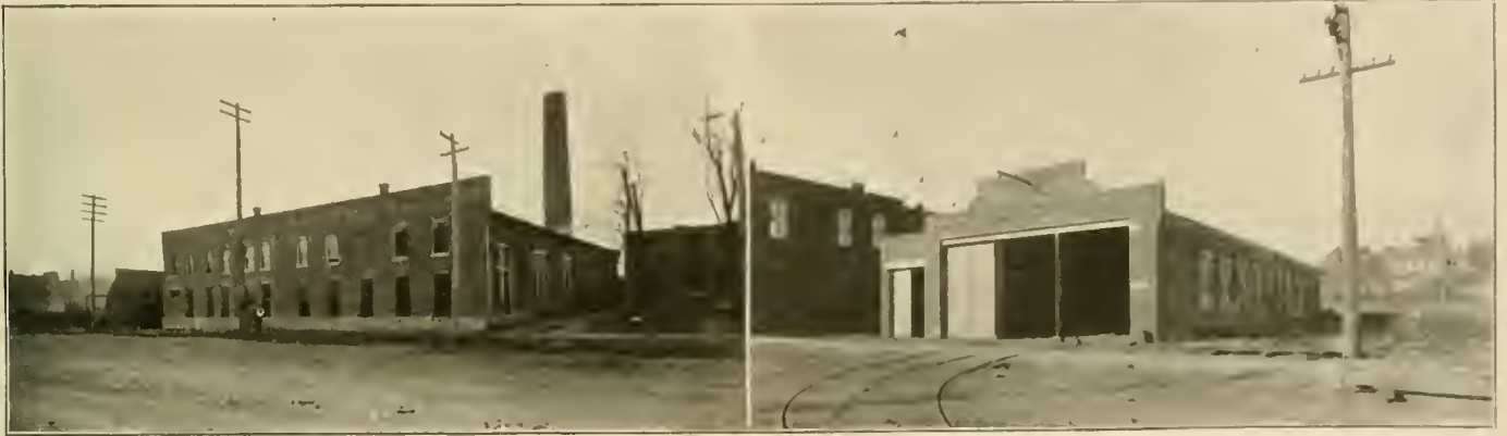
FIG. 1. POWER STATION AND CAR BARN AT ATCHISON, KAS. FIG. 2.
