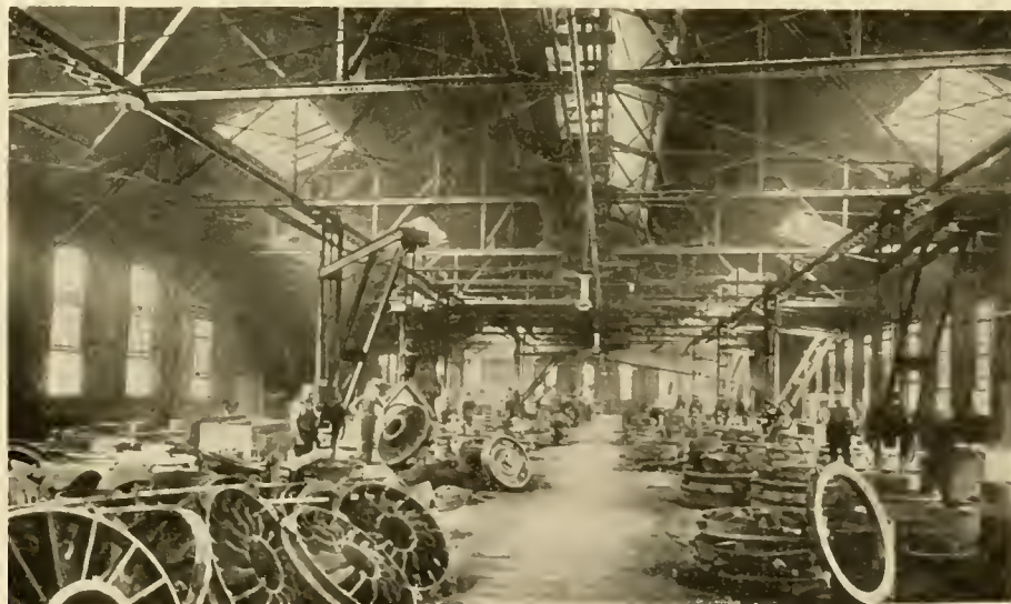
FIG. 2. INTERIOR OF MAIN FOUNDRY.
