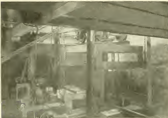
VIEW IN BASEMENT.
