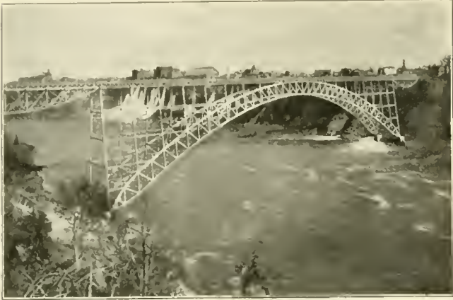
FIG. 2—NEW STEEL ARCH BRIDGE.
