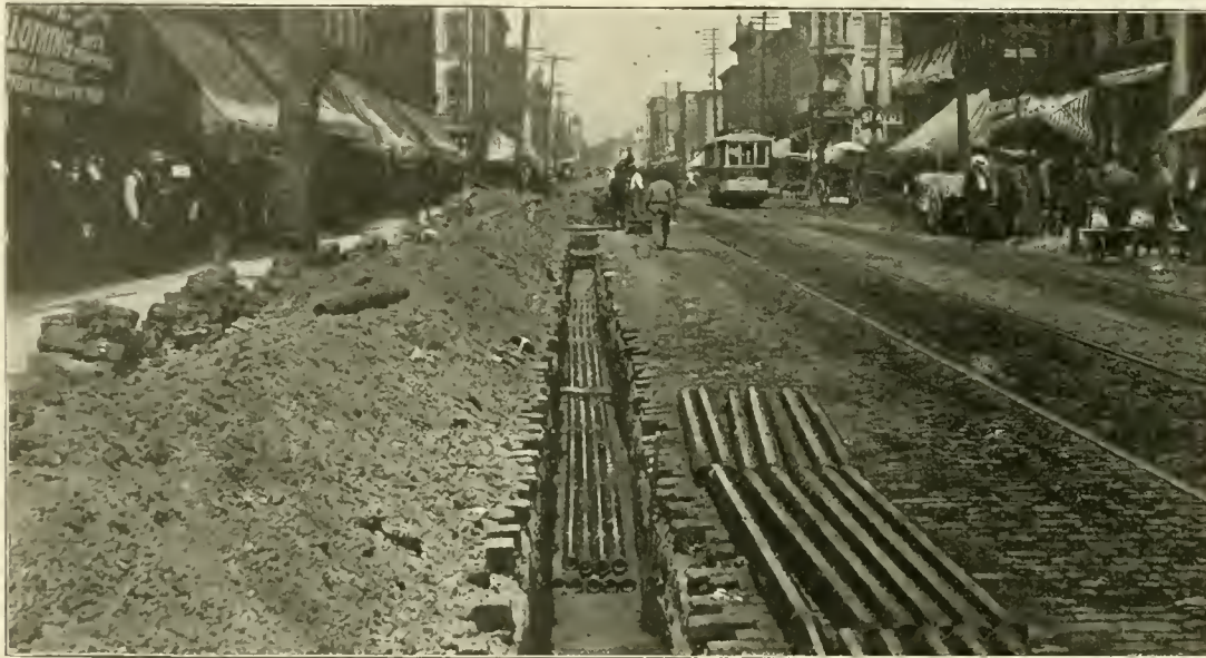
MONROE ST., TOLEDO, SHOWING TRENCH WITH NINE DUCTS.
