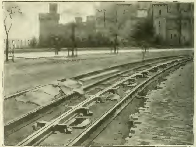
CABLE TRACK CONSTRUCTION, EDINBURGH.
