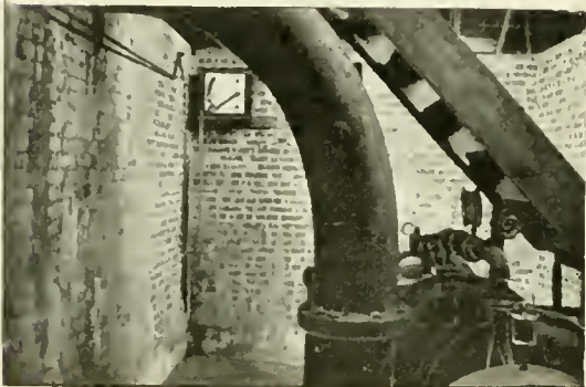
NEGATIVE LEADS ON LARGE GENERATOR.
