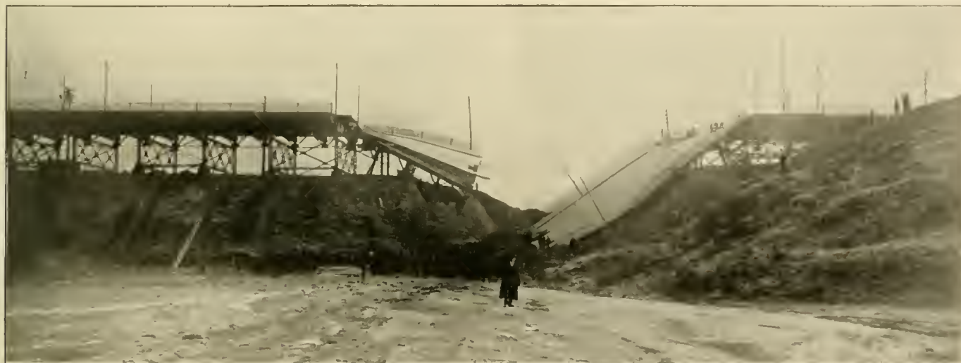
WILLSON AVENUE VIADUCT, CLEVELAND.
