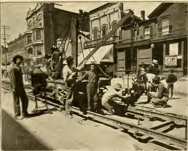
RIVETING JOINTS.
