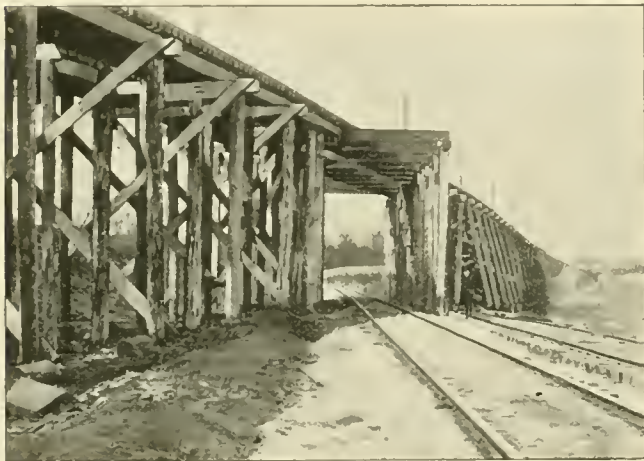
CROSSING OVER AIR LINE TRACKS.
