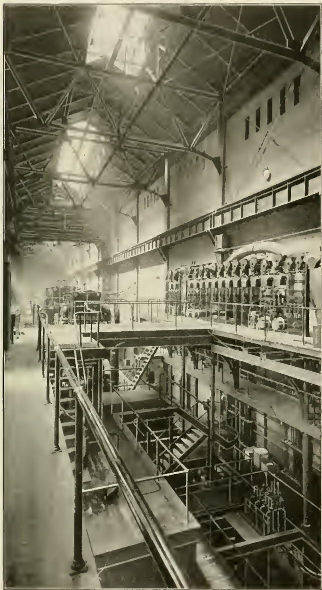
INTERIOR OF METROPOLITAN POWER HOUSE.
