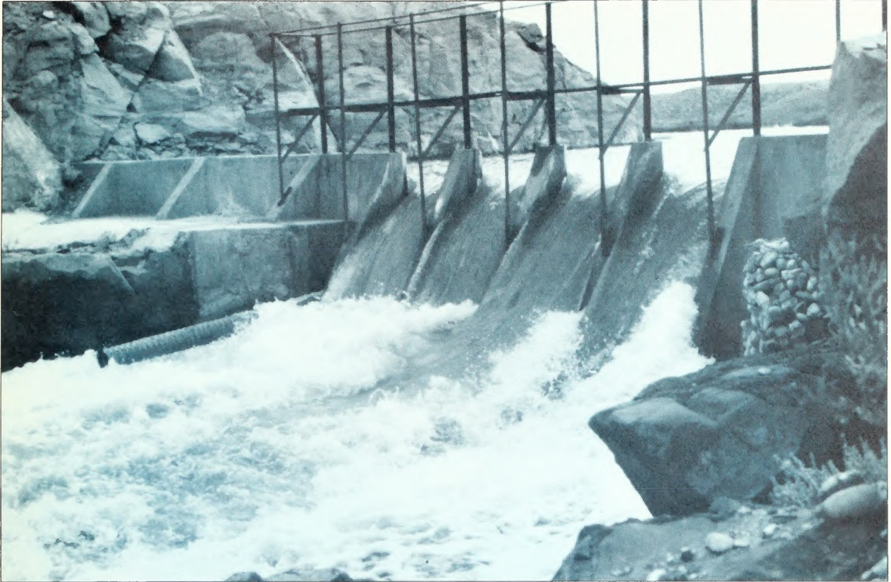
Water Diversion Dam
