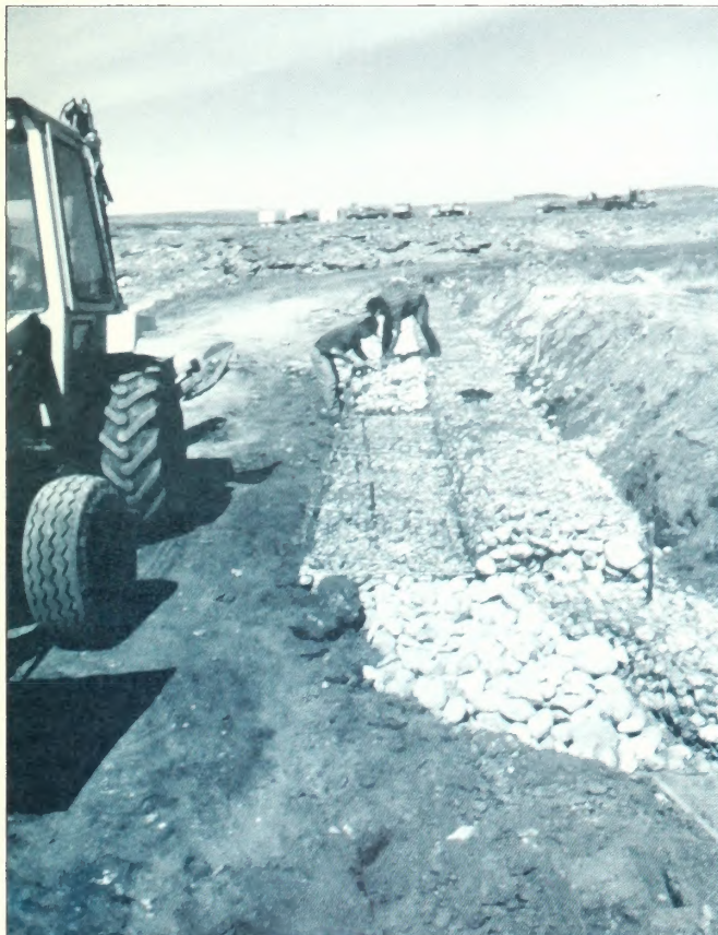
Building Rock-Lined Drain
