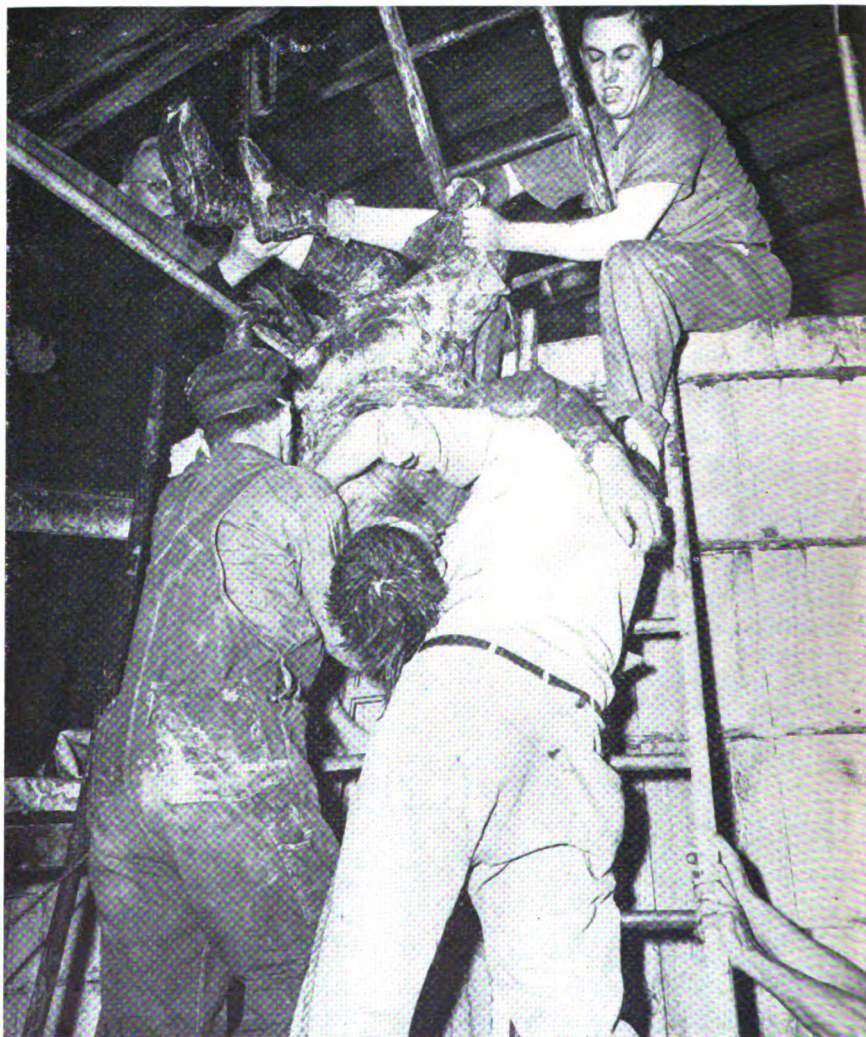
An unconscious worker, overcome by hydrogen sulfide, is removed from a wooden gluten vat. Photograph by courtesy of Indianapolis Star.
