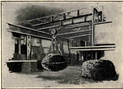
Fig. 7.—Aloxite ingots as they come from the furnace.
