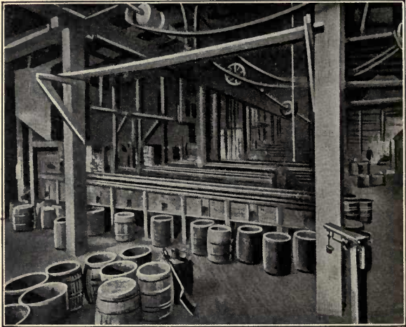
Fig. 4.—Screening machines used in grading Carborundum.
