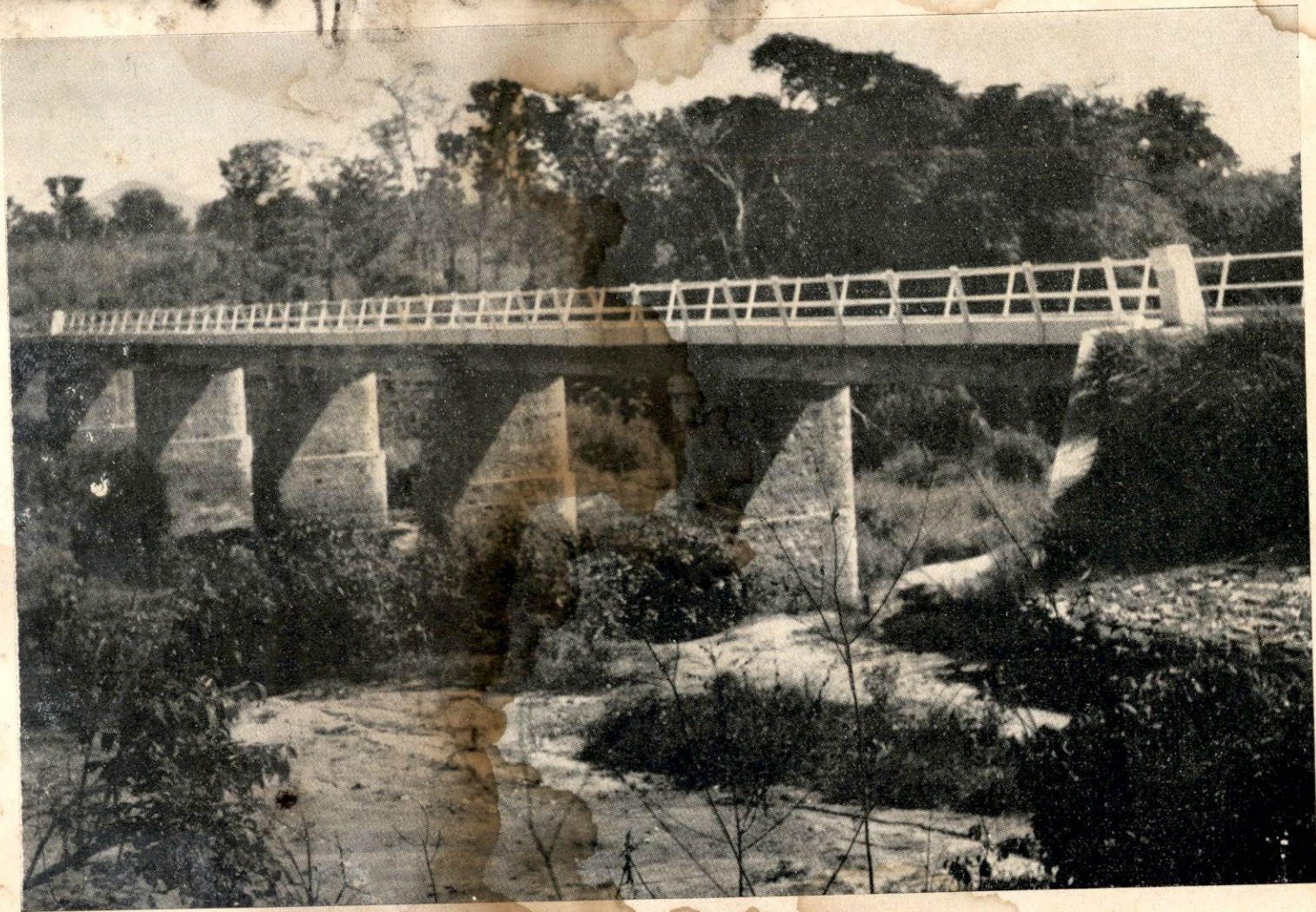
YOLA-WUKARI ROAD—SIX 40 FEET STANDARD SPANS CROSSING RIVER FAN MANGA 130 MILES FROM YOLA
