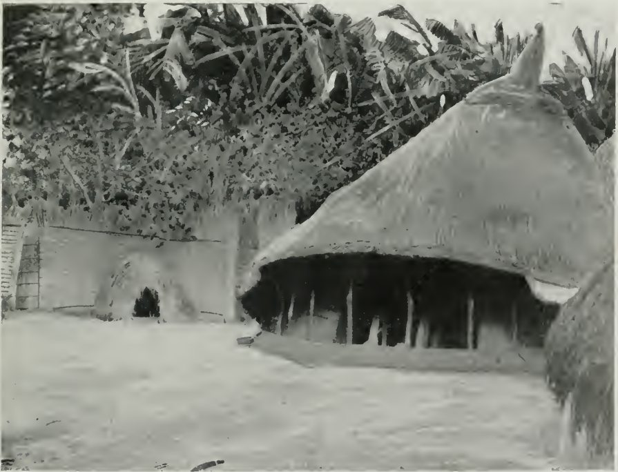
367. A HOUSE AND COURTYARD, UGANDA.
