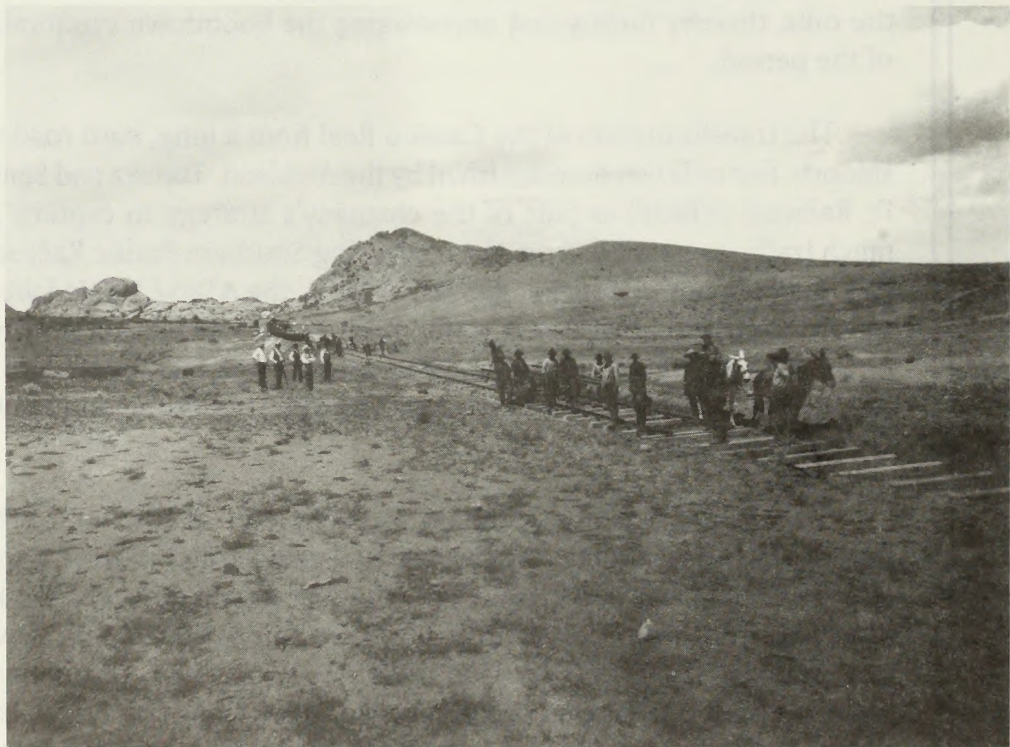
Figure 55. Laying track, courtesy of National Archives, negative no. 92-F-79B-21.
