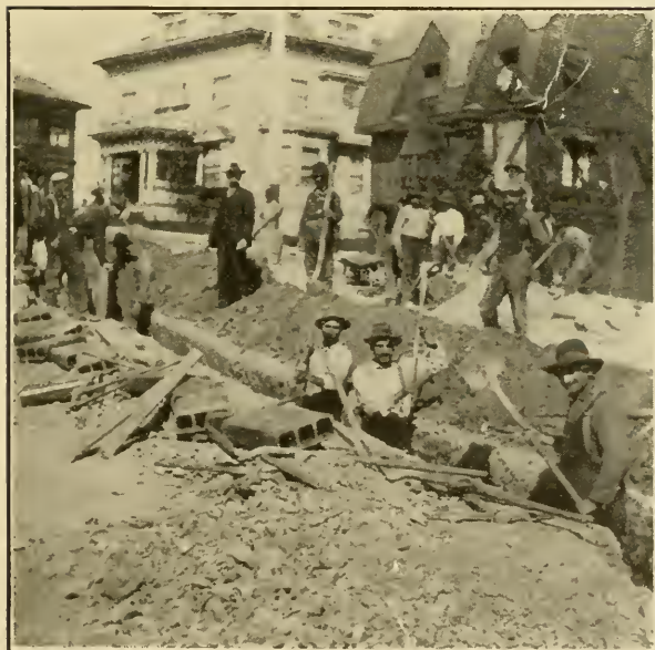
Trench Construction Work
