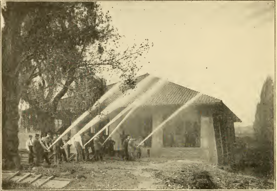
Pumping Station near Lake Merritt
