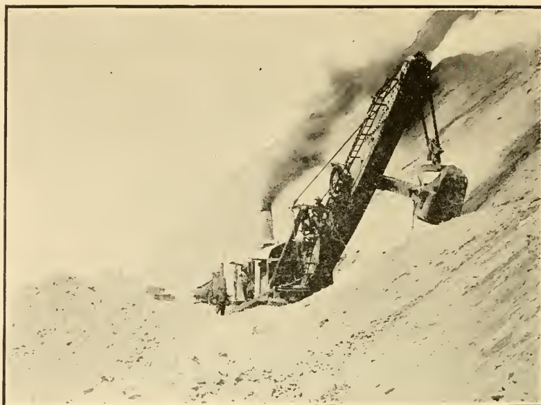
Steam Shovel at Work, Ocean Shore Road. Ransome-Crummey Construction Co.
