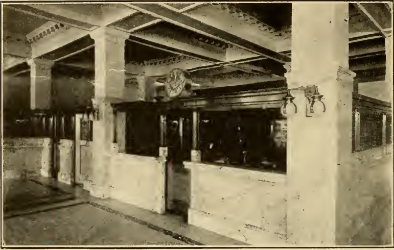
Interior View, Central National Bank
