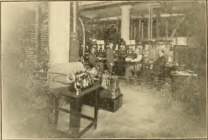
Terminal Room, Showing Wire Chief's Test Board
