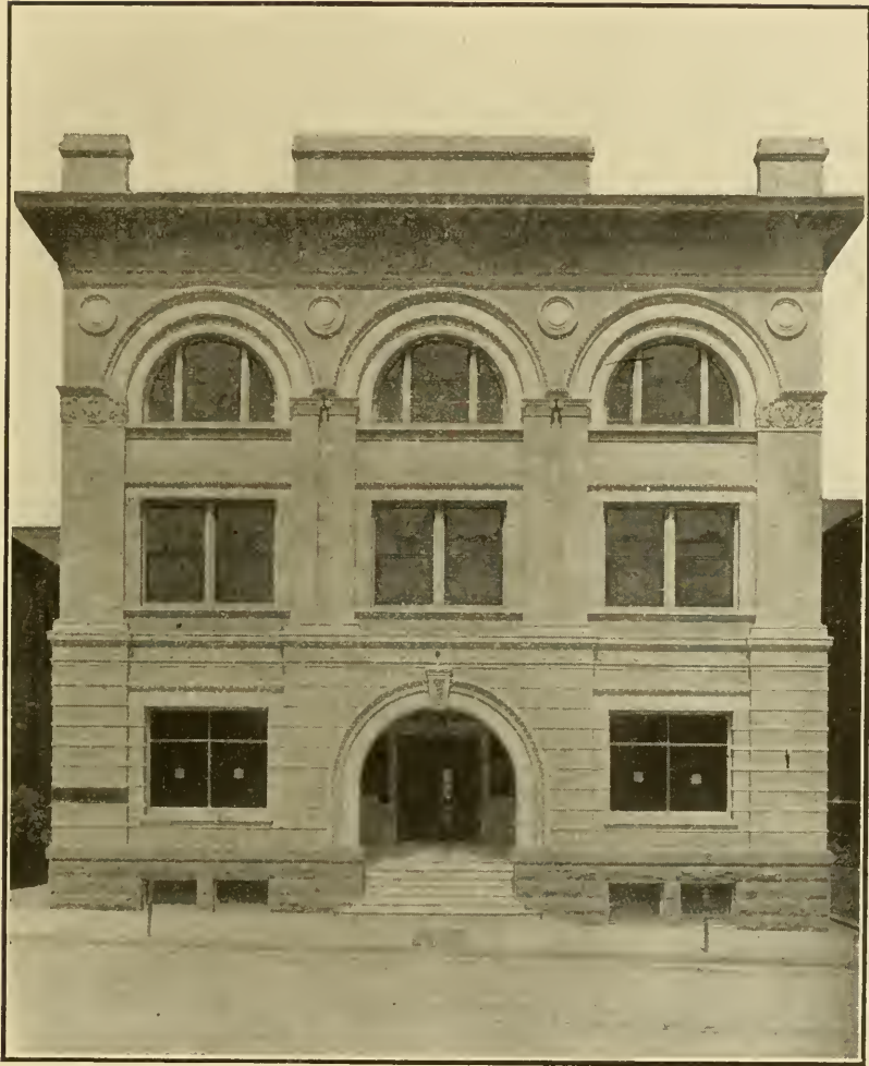
Main Office Bay Cities Home Telephone Company
