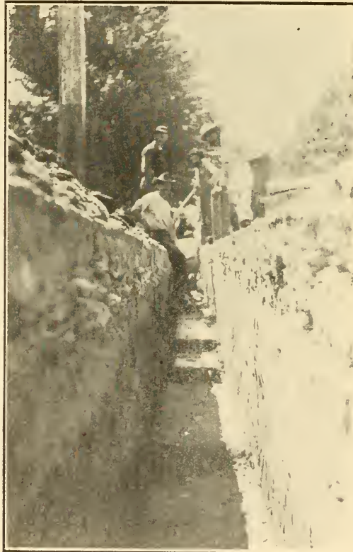
Laying an Underground Trench
