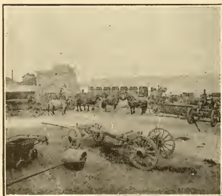
Stable Yard and Warehouse, 26th and Poplar Sts.
