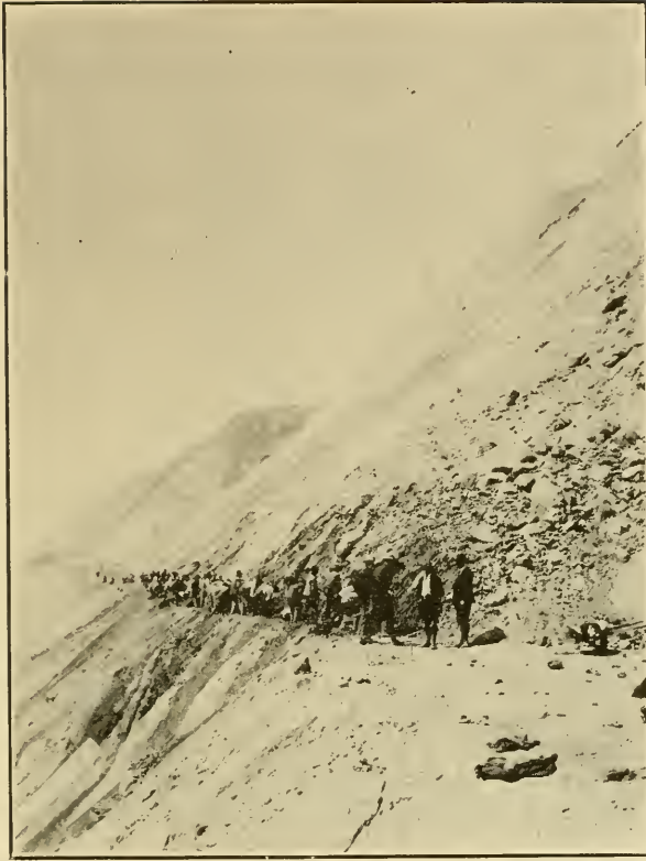
Gang at Work Grading for Ocean Shore Road. Ransome-Crummey Co.
