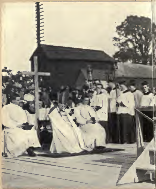
AN OPEN AIR SERVICE The occasion was the laying of the Foundation
