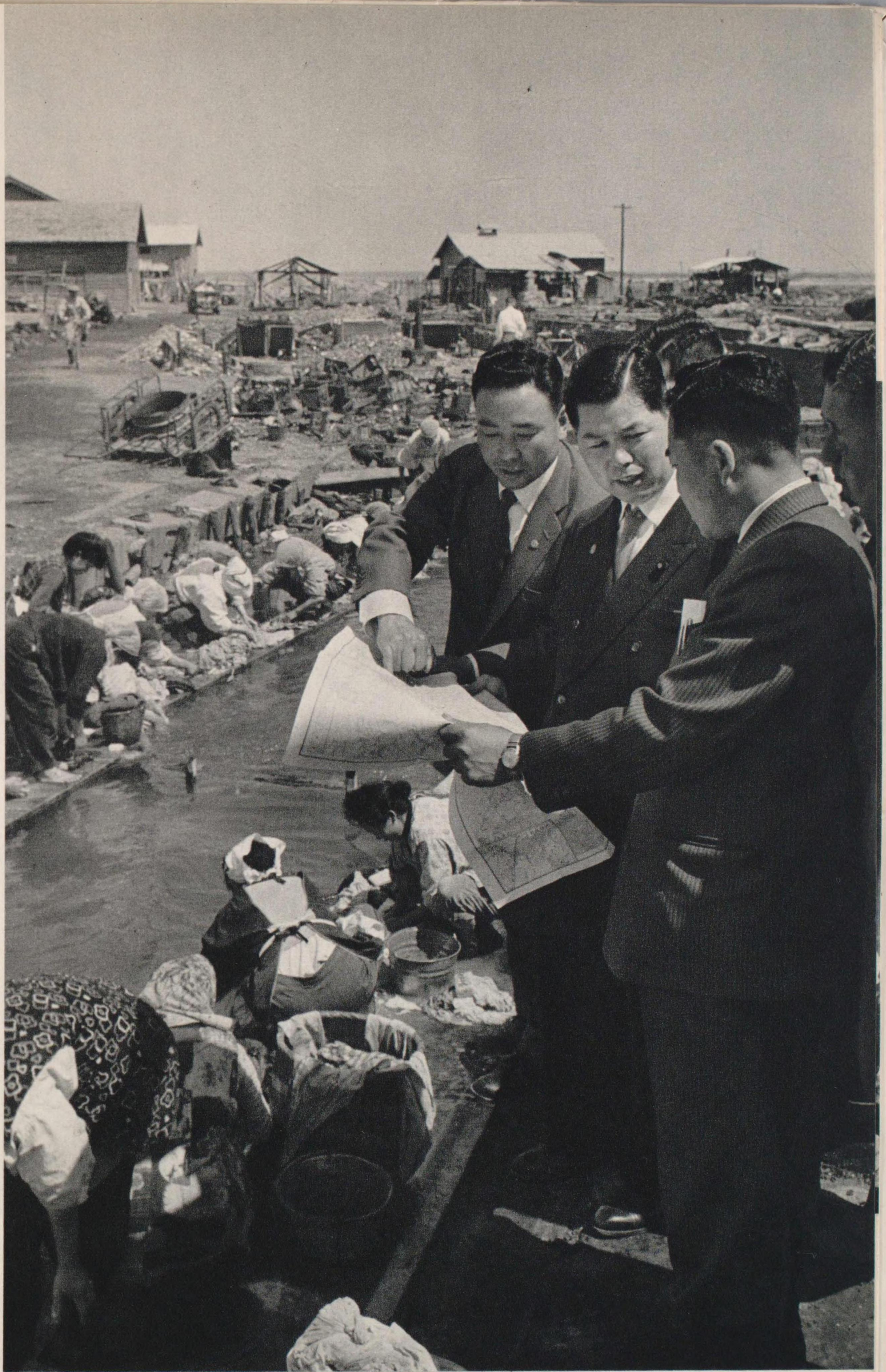
When an accident happens they hurry to the scene to help. Mr. Tsuji is making a field inspection.
