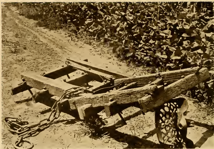
52. A HOME-MADE SPIKE-TOOTH HARROW, IN TWO SECTIONS
