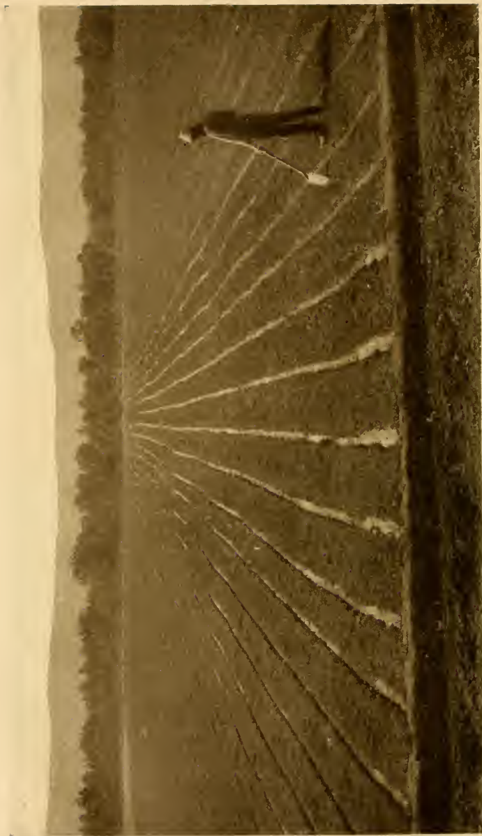
81. IRRIGATING ALFALFA BY FURROW SYSTEM, YAKIMA VALLEY, WASHINGTON
