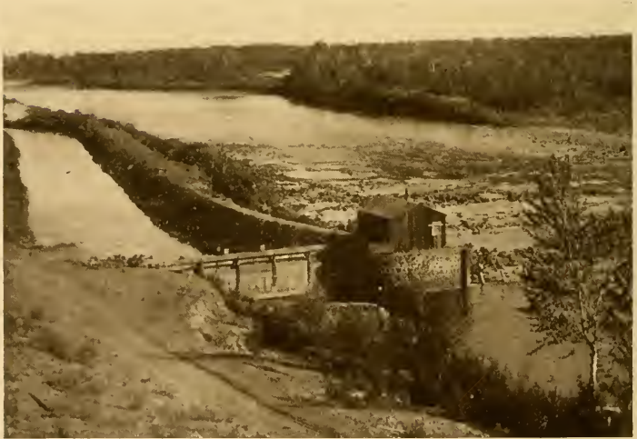
81. THE INTAKE OF THE SUNNYSIDE CANAL, YAKIMA VALLEY, WASHINGTON Note the head-gate. These large canals are usually built by corporations or partnerships of farmers
