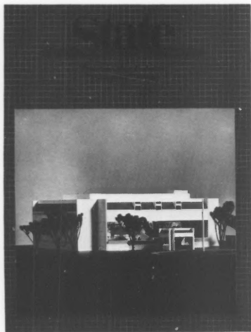
THE COVER —This model, which at first glance doesn't appear to have security features, does in fact have reinforced recessed windows and a single main entrance, as well as other safeguards that aren't obvious. See interview with Robert E. Lamb starting on Page 4.
