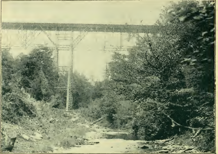
MILL CREEK BRIDGE—118 FT., Dansville, N. Y.
