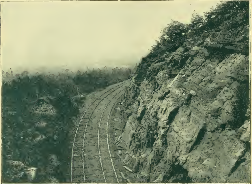
NORTHERN APPROACH TO PARADISE TUNNEL.
