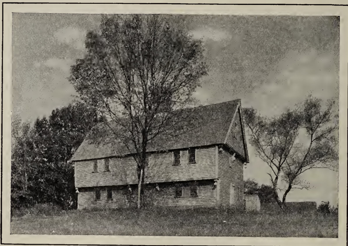
THE PARSON CAPEN HOUSE, TOPSFIELD, MASSACHUSETTS. BUILT 1683
