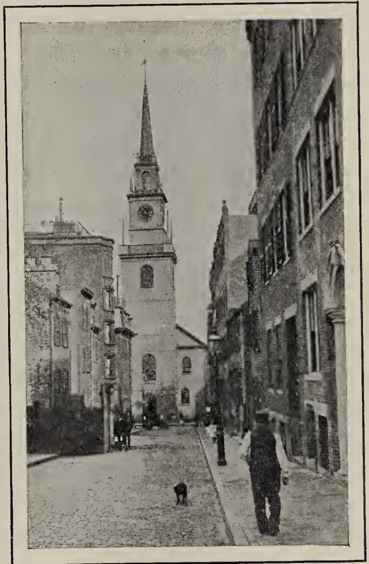
EXTERIOR OF OLD NEW ENGLAND CHURCH
