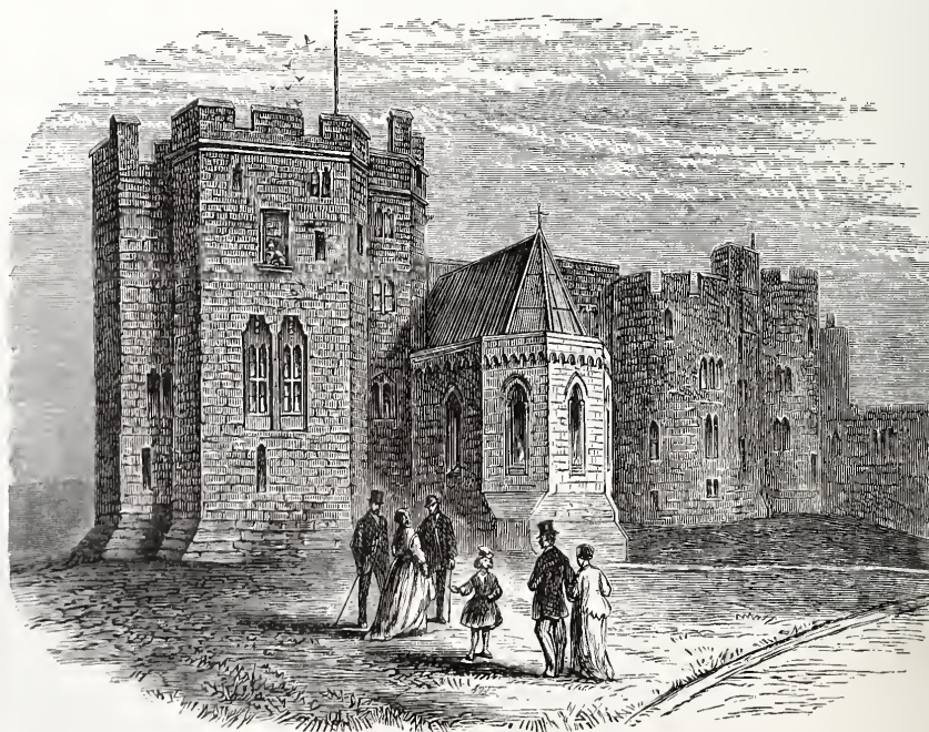
THE PRUDHOE TOWER AND CHAPEL.
