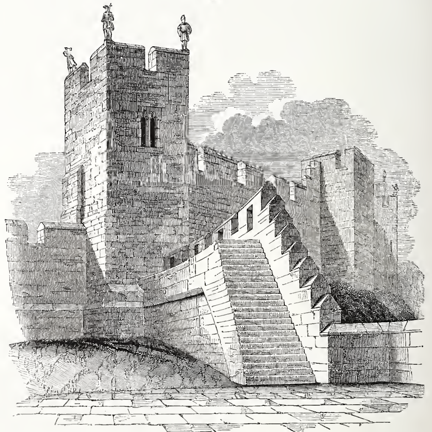
THE ARMOURER'S TOWER.
