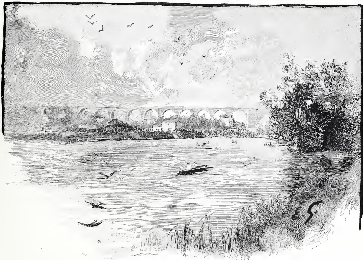
The Viaduct of Nogent.
