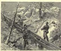
particles of gold as they are borne along by the current of water. The sluice may be of any width or length corre-aponding with the amount of material to be handled; but the supply of water must be sufficiently abundant, and the topographic conditions favorable, especially as re-gards the disposal of the tailings.
