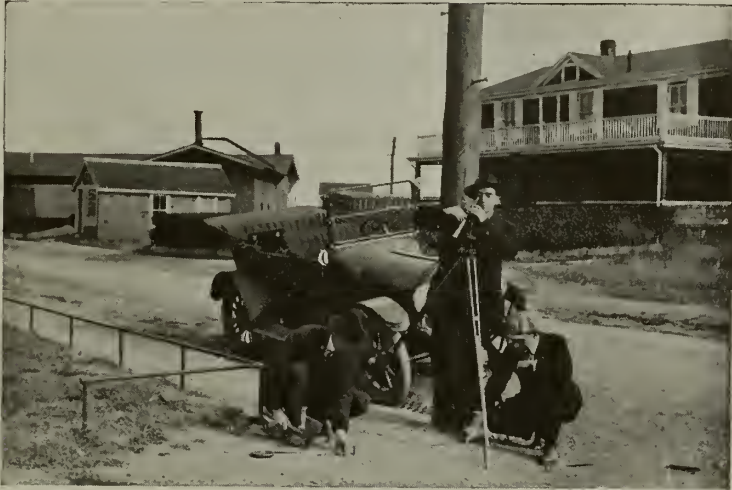
Locating Edge Stones Whitman and Howard, Civil Engineers
