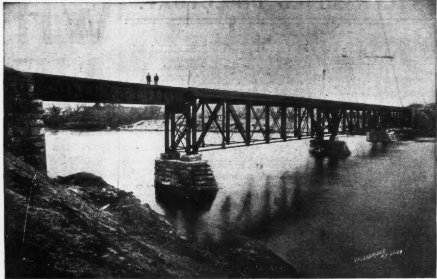
BRIDGE OVER THE MERRIMAC RIVER AT CONCORD, N. H.
