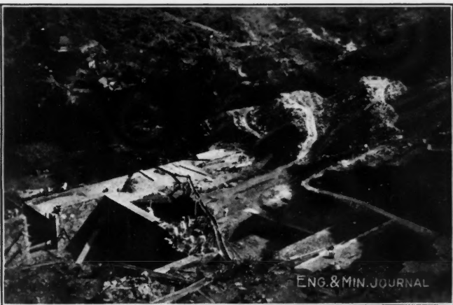
WILFLEY TABLE FOUNDATIONS AND MILL FOUNDATIONS FROM CONCRETE MIXING PLANT The Cinco Minas mill was recently completed and has been built despite the political strife in Mexico.
