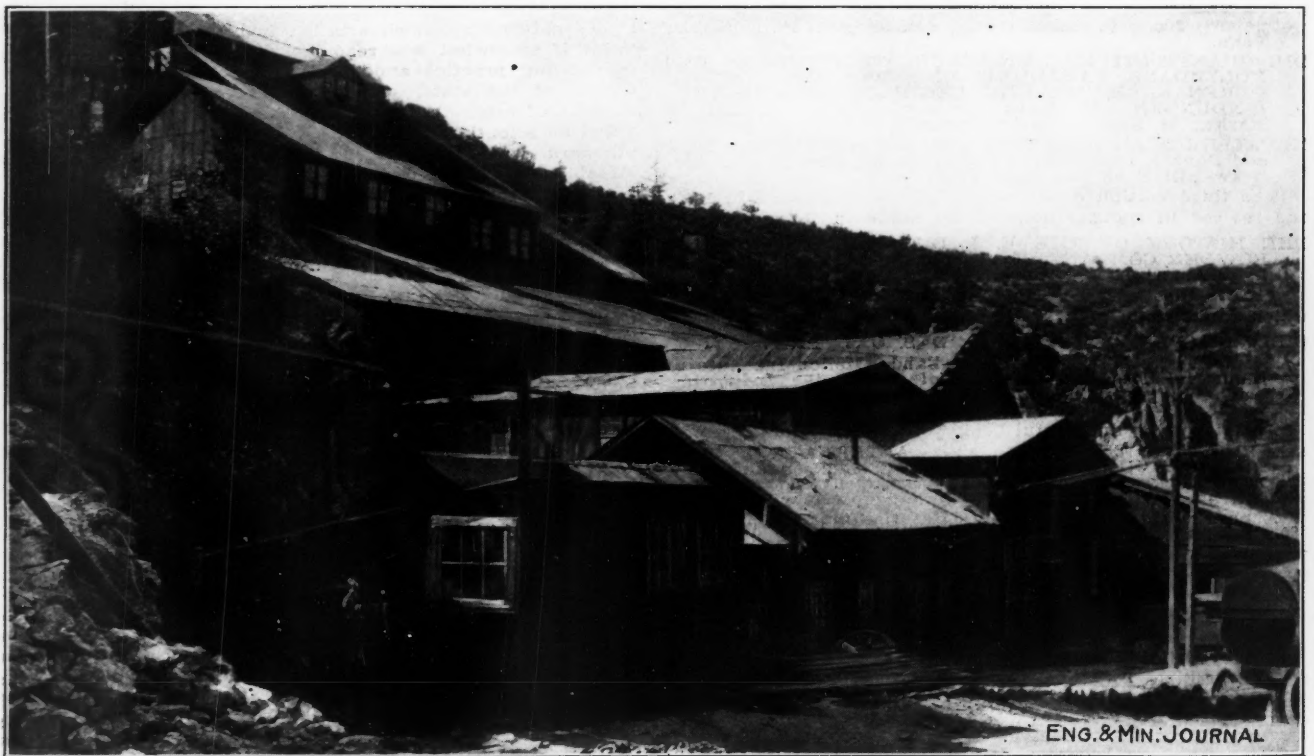
THE ERNESTINE MILL IN THE MOGOLLON DISTRICT IN NEW MEXICO
