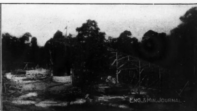
COMPLETED FRAME OF MILL
