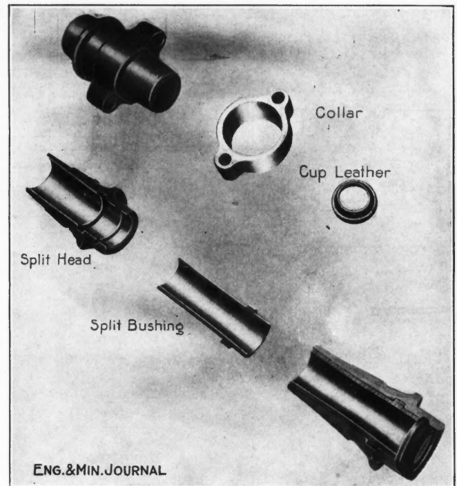
INGERSOLL-RAND BUTTERFLY-VALVE PISTON MACHINE FRONT HEAD
