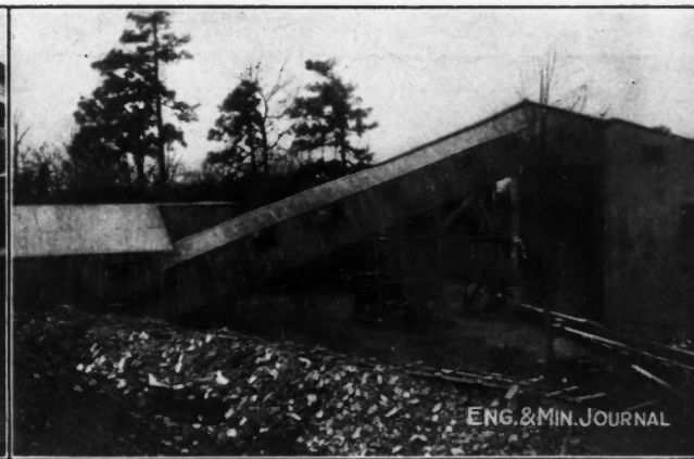
BACK OF THE MILL, SHOWING INCLINE
