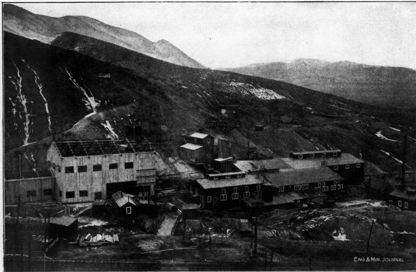
The plant under construction. BUTTE DULUTH MINING CO., BUTTE, MONT.
