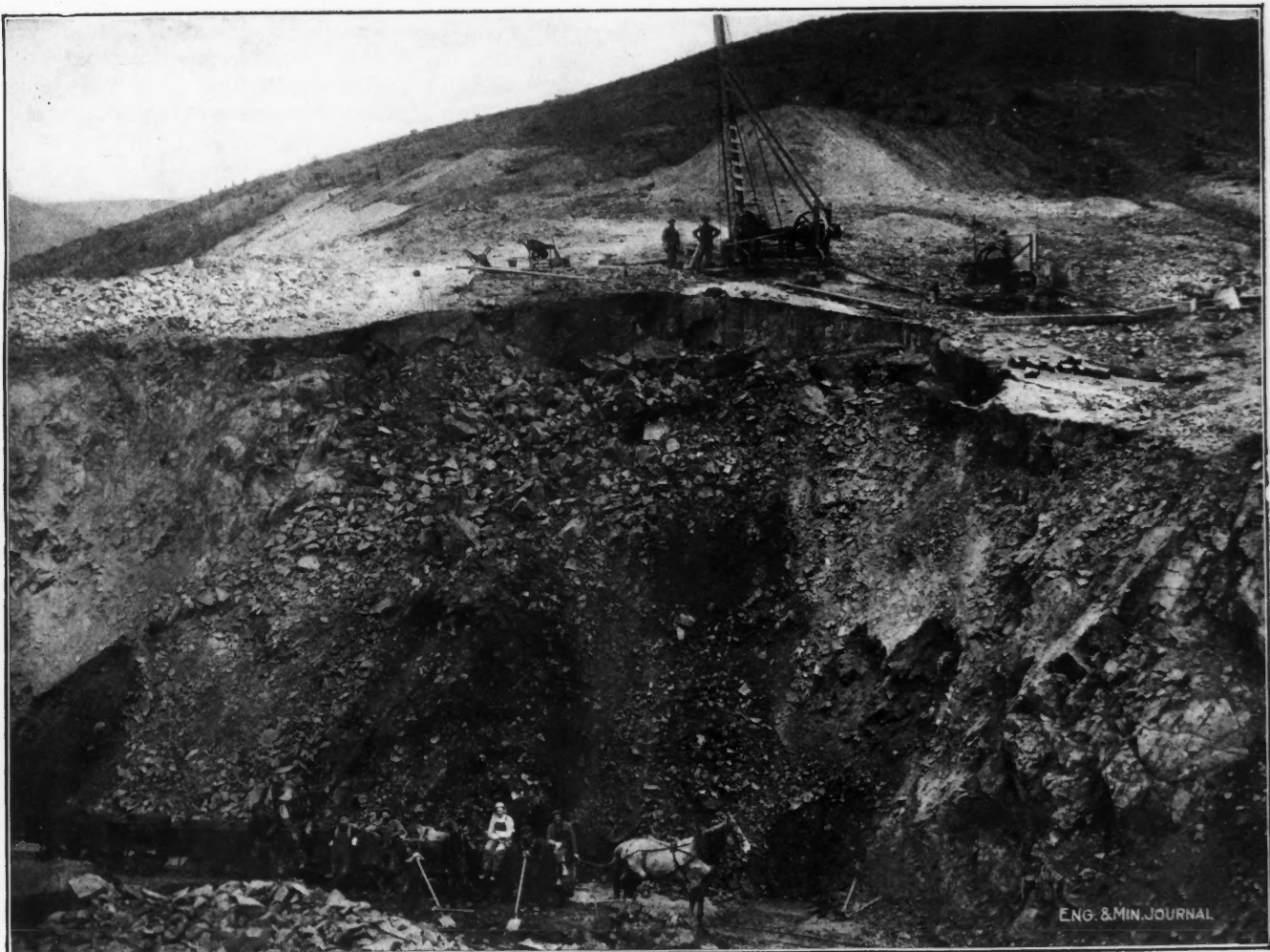
Putting down shot holes in opencut pit. BUTTE DULUTH MINING Co.
