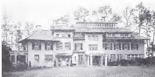
ENTRANCE VIEW OF DE LANOY HOUSE
