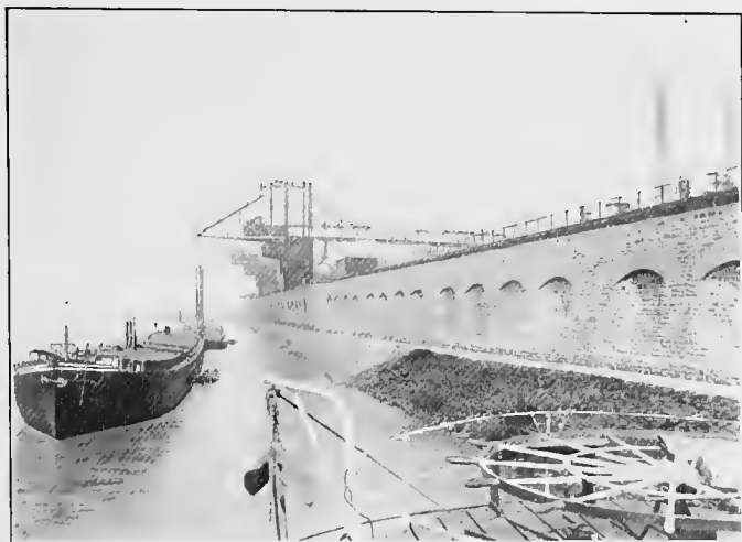
HOISTS DISCHARGING SPANISH IRON ORE THAT HAS COME UP FROM ROTTERDAM BY BARGE IN THE BACKGROUND ARE BLAST FURNACES. RUHRORT
