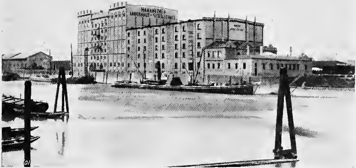
GRAIN ELEVATOR AND WAREHOUSE IN A BASIN OF THE MANNHEIM HARBOR
