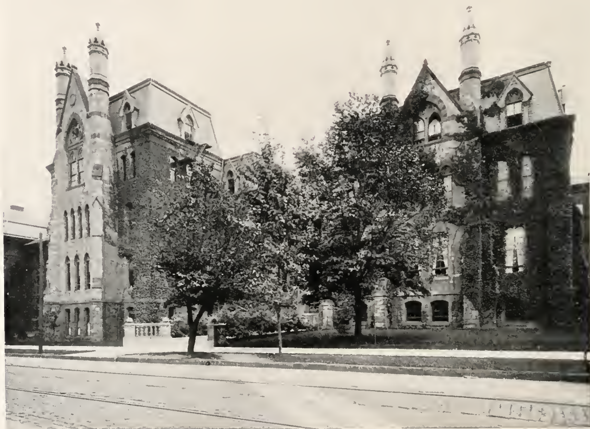
MAIN HOSPITAL BUILDINGS
