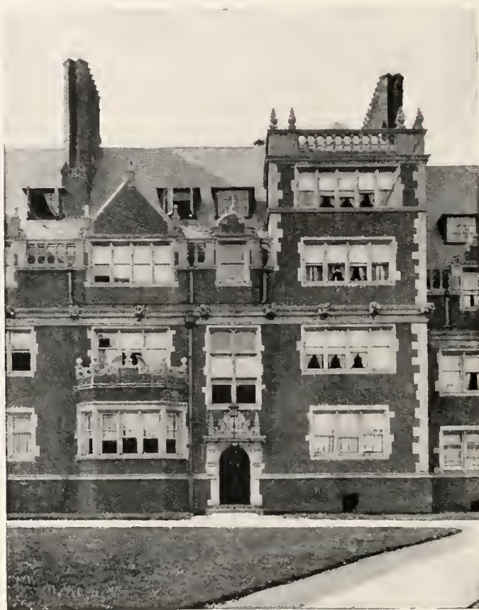
DETAIL OF DORMITORIES
