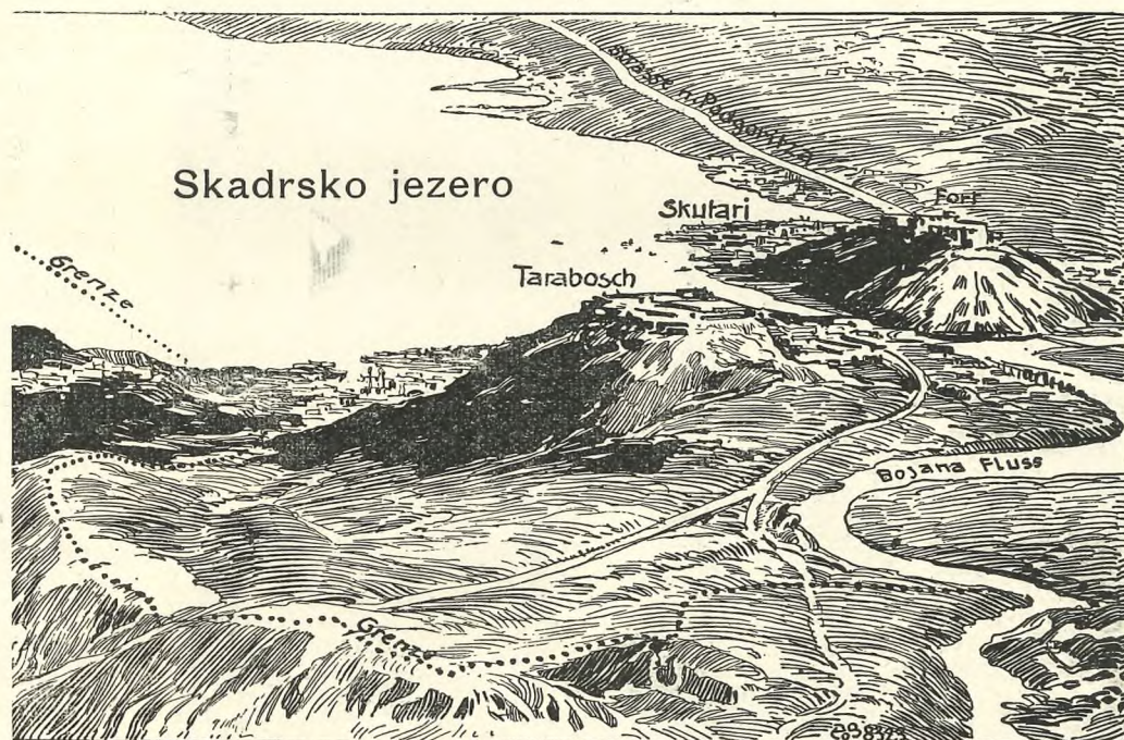
Skader in Taraboš.
