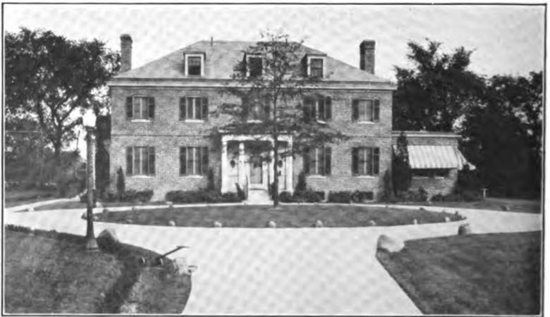
THE PRINCIPAL'S HOUSE
