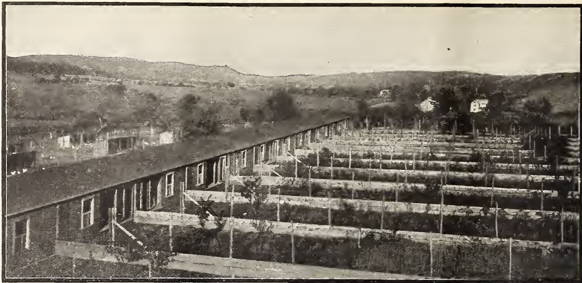
PLAINFIELD POULTRY FARM—Laying-house for Hens. Length 240 feet.
