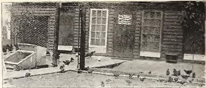
Section of Poultry House of W. T. Wittman, Allentown, Pa. See page 273.
