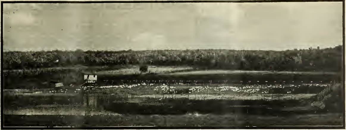
PLAINFIELD POULTRY FARM—Main Laying-house for Ducks. Length 400 feet. Feed House Attached.
