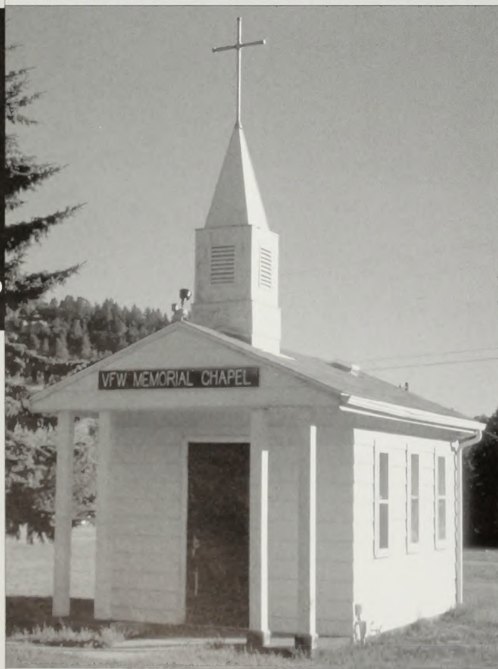
World War II Memorial Chapel at the Fort Meade Post Cemetery in Montana's Fort Meade Recreation Area.
