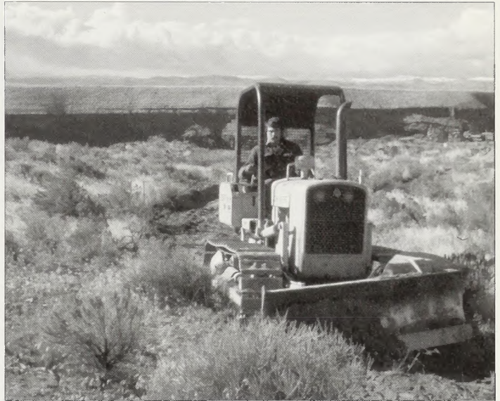
Rental equipment being used in Idaho.
