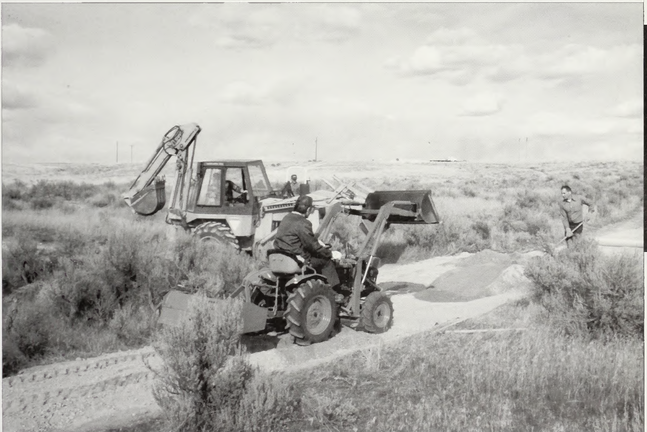
Rental equipment being used for road maintenance in Idaho.
