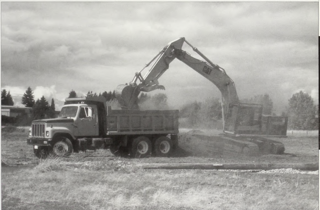
Road maintenance crew at work in Oregon.
