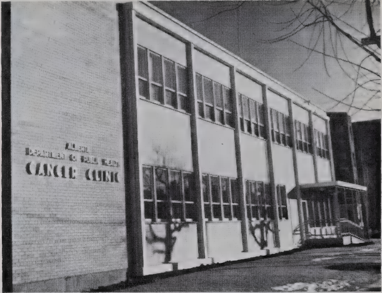
The Cancer Clinic, shown following completion last autumn.
