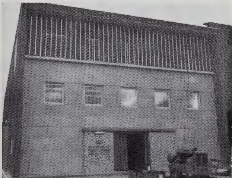
The new Public Works Power Plant (South).
