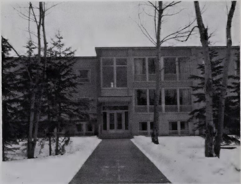
The Nurses' Residence at Ponoka Mental Hospital, shown at completion.
