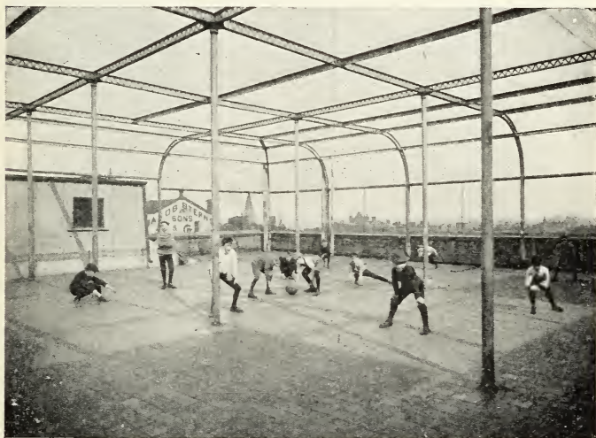
Boys' Roof-Playground, Public School 126, Brooklyn. Possibilities for Roof-Gardening.
