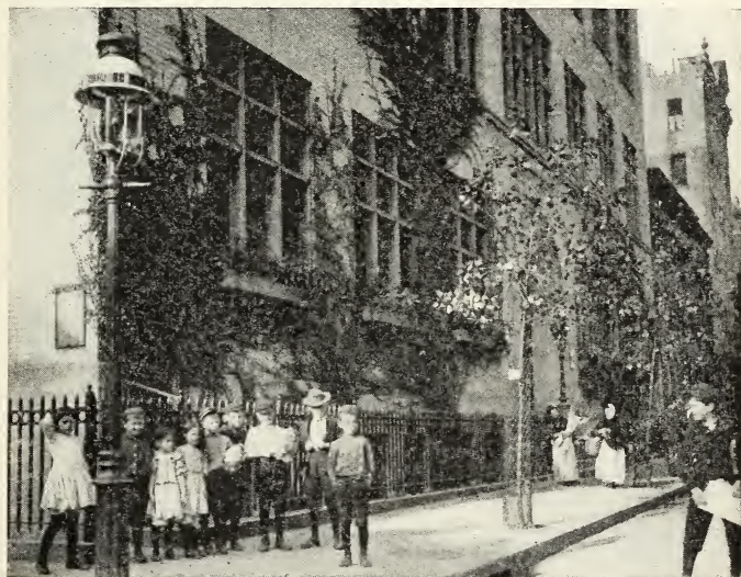
Window-Gardens: the Alfred Corning Clark Neighborhood House, Rivington Street, New York City.
