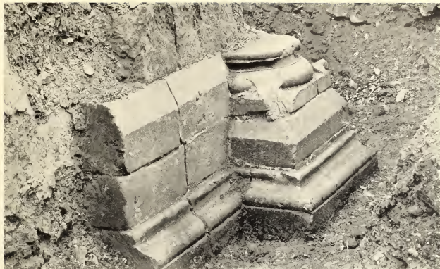
PIER OF EASTERN ARCADE OF NORTH TRANSEPT.
