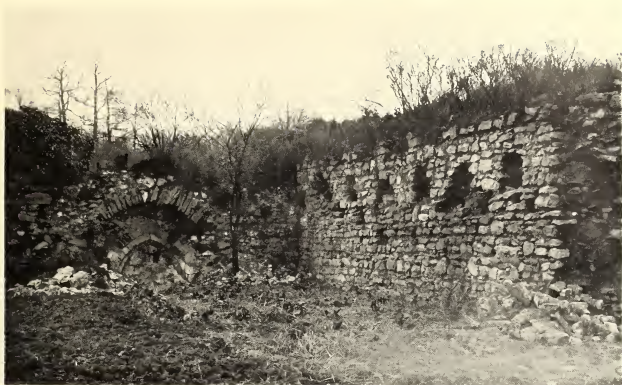
NORTH WALL OF NAVE, EXTERIOR.
