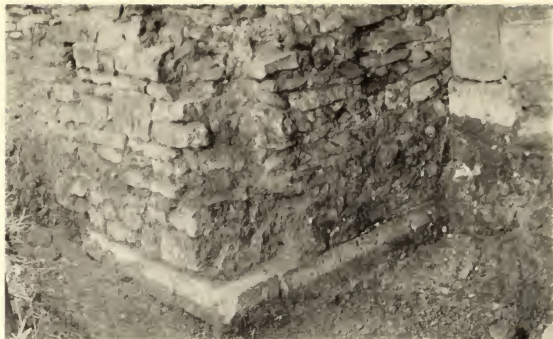
NORTH-WEST BUTTRESS OF NAVE.
