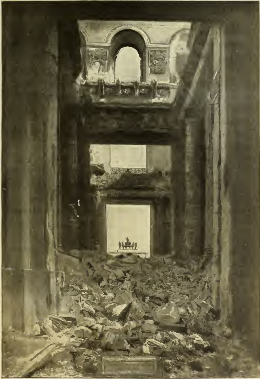
THE RUINS OF THE TUILERIES, MAY 1877.
