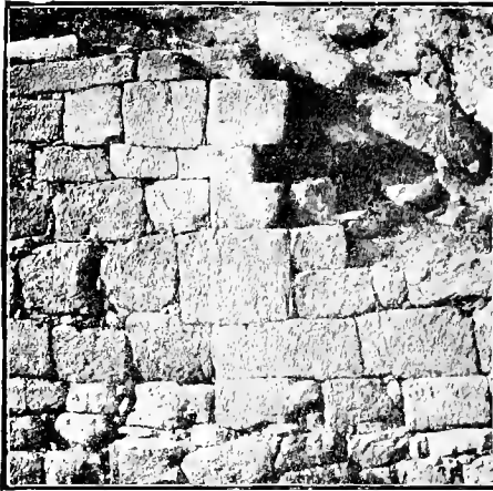
FIG. 9. RETAINING WALL OF VI M
