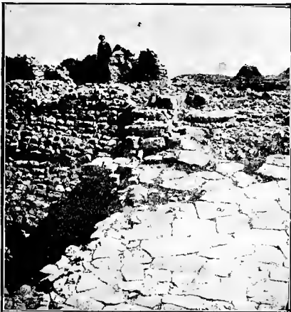
FIG. 6. PAVED RAMP AT GATE FM (II STRATUM)
