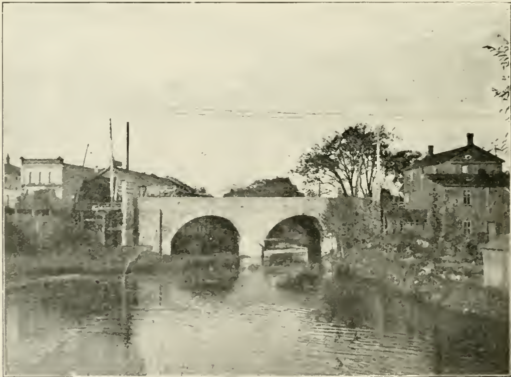
STONE ARCH BRIDGE, STRATFORD.
