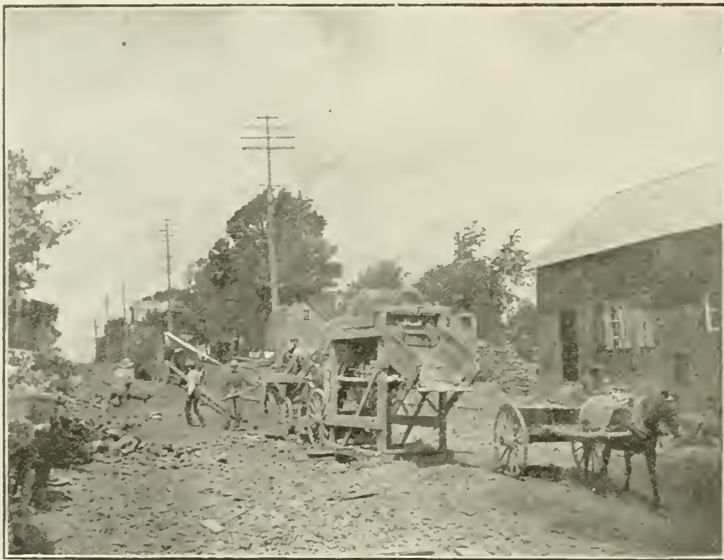
CRUSHING STONE AT CARLETON PLACE.
