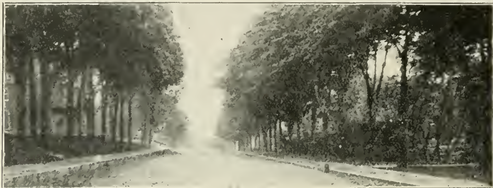
A MACADAM STREET IN BROCKVILLE.
