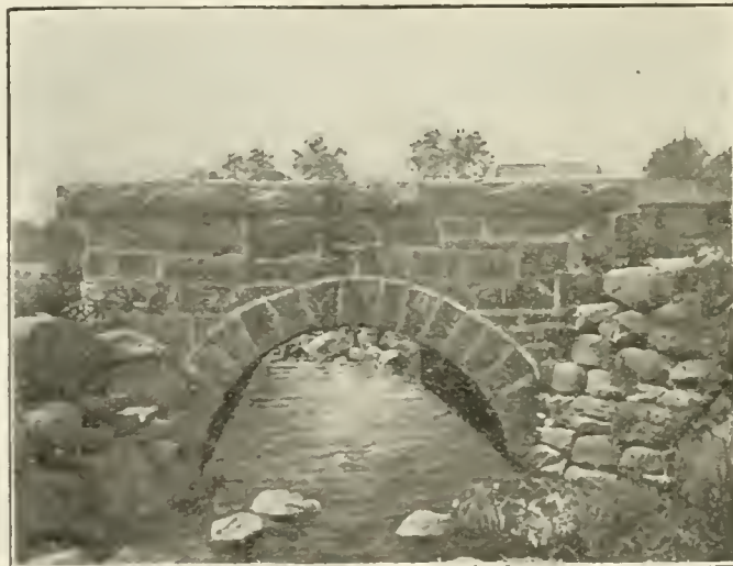
STONE CULVERT, CORNWALL.
