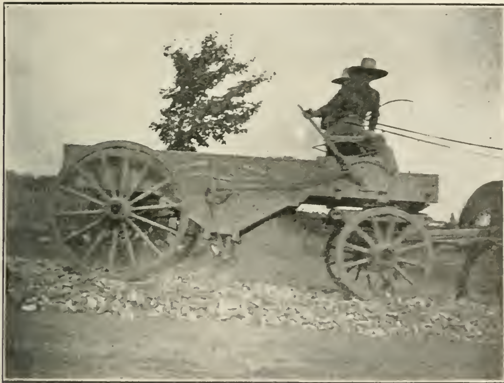
HAULING AND SPREADING BROKEN STONE IN THE RIGHT WAY.
