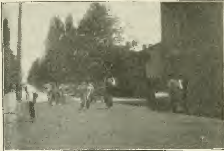
FINISHING THE SURFACE WITH TARRED GRAVEL.
