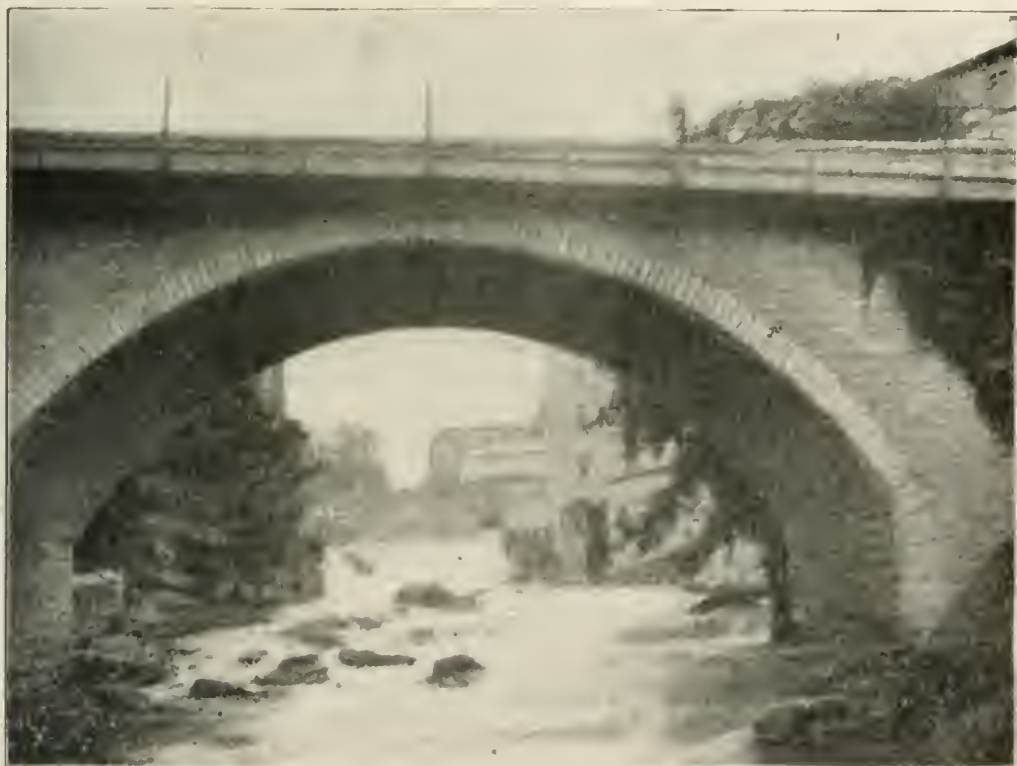
STONE ARCH CULVERT, ALMONTE.
