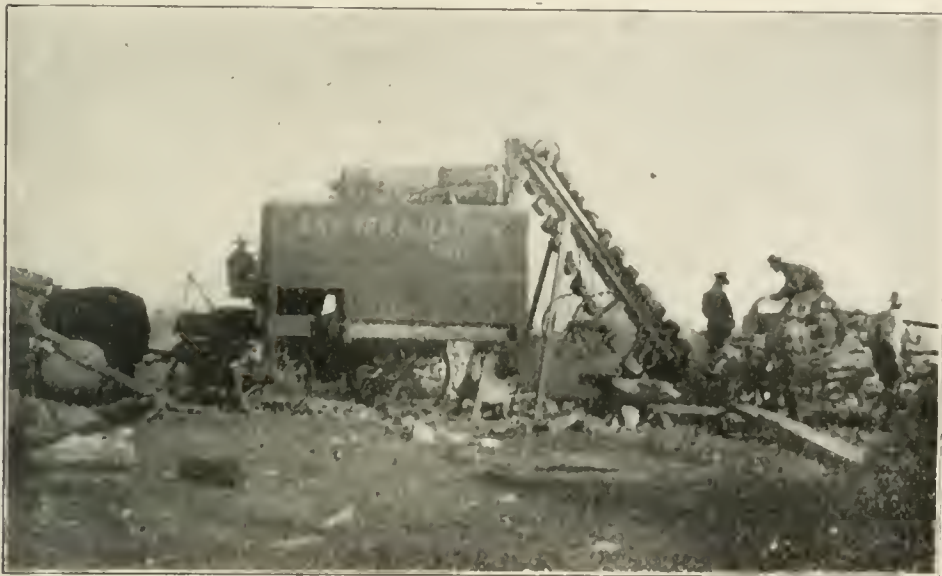
THE CRUSHER AND SCREEN ATTACHMENT. Loading from the bins.
