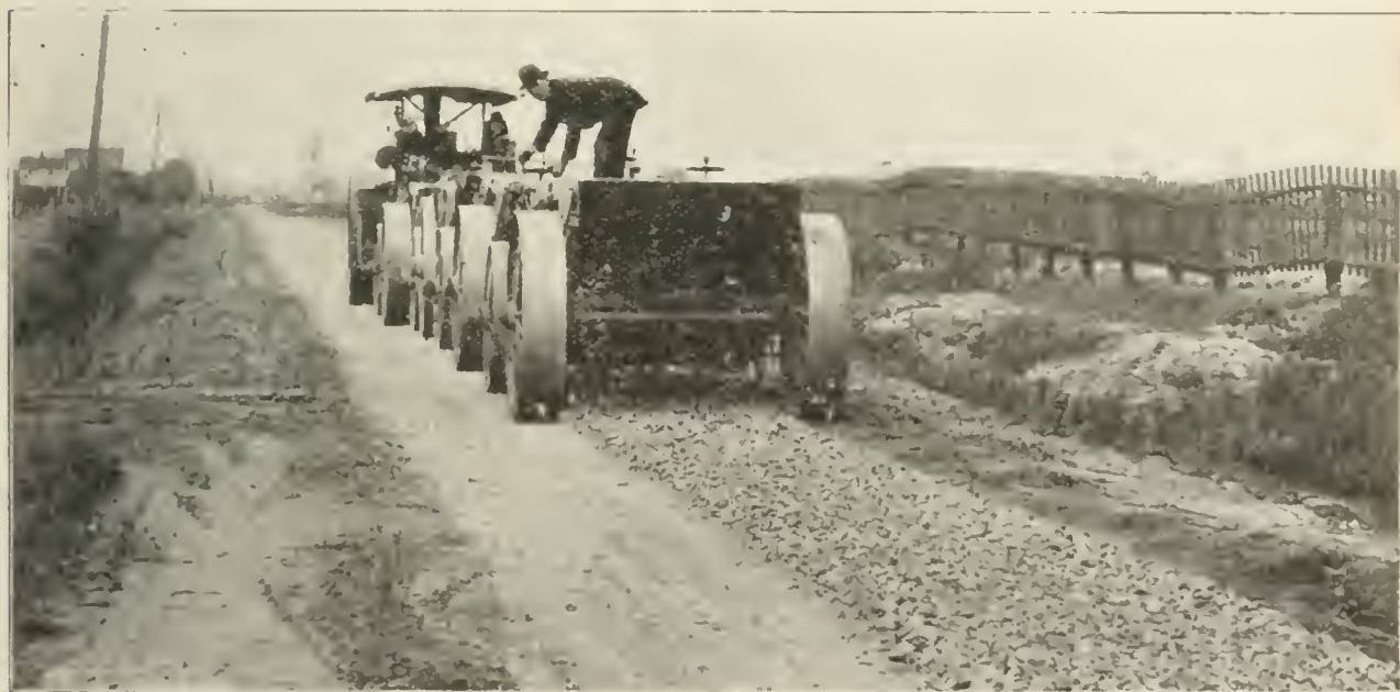
HOW STONE SHOULD BE SPREAD.
