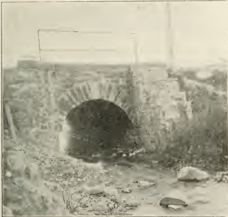
ONE OF THE STONE CULVERTS AT INGERSOLL.
