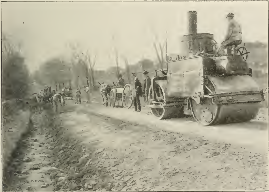
A STEAM ROAD ROLLER AT WORK.
