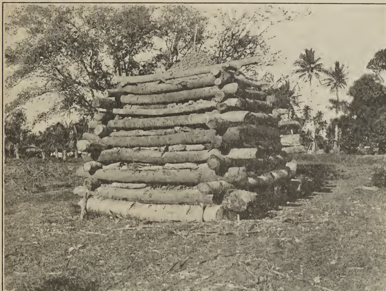
FIG. 3.—Native lime kiln before burning
