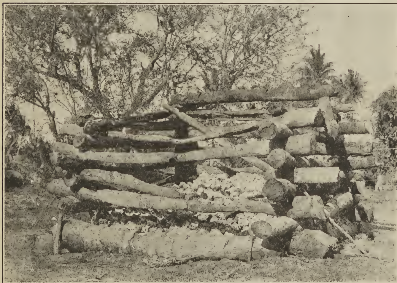
FIG. 4.—Native lime kiln after burning
