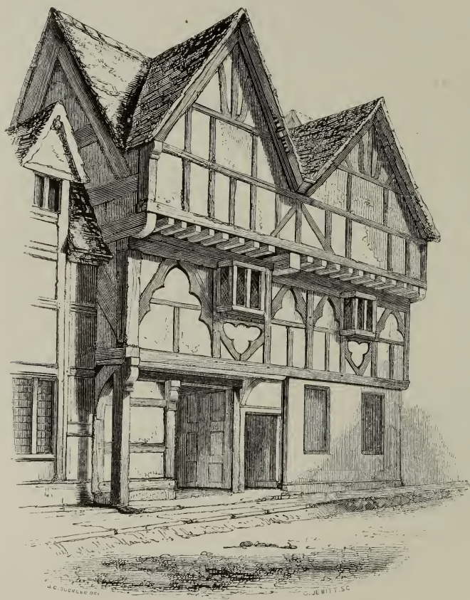
TIMBER HOUSE AT TAMWORTH.
