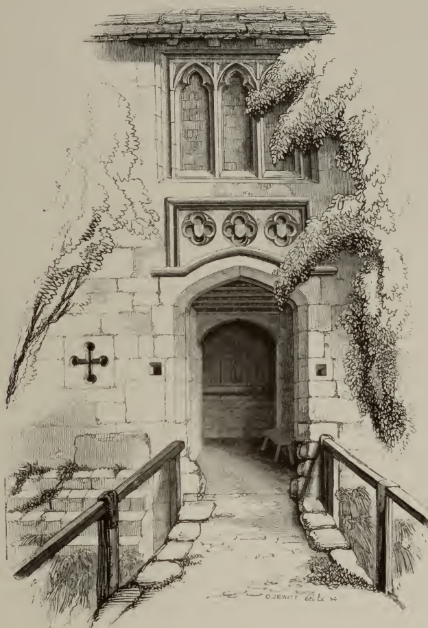
ENTRANCE TO THE MOAT HOUSE, APPLEBY, LEICESTERSHIRE.
