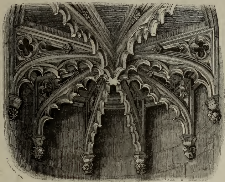
Stone Roof at the top of the Newel Staircase.
