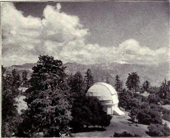
FIG. 51.—Dome of 60-inch Reflector.
