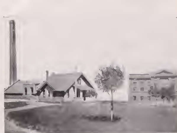
CENTRAL HEATING PLANT
