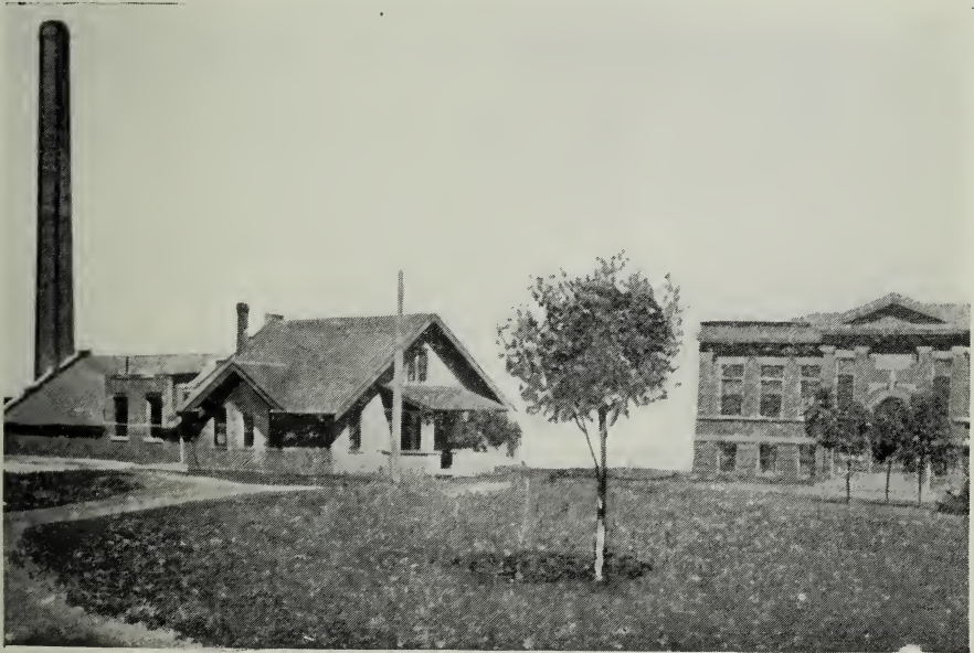
CENTRAL HEATING PLANT
