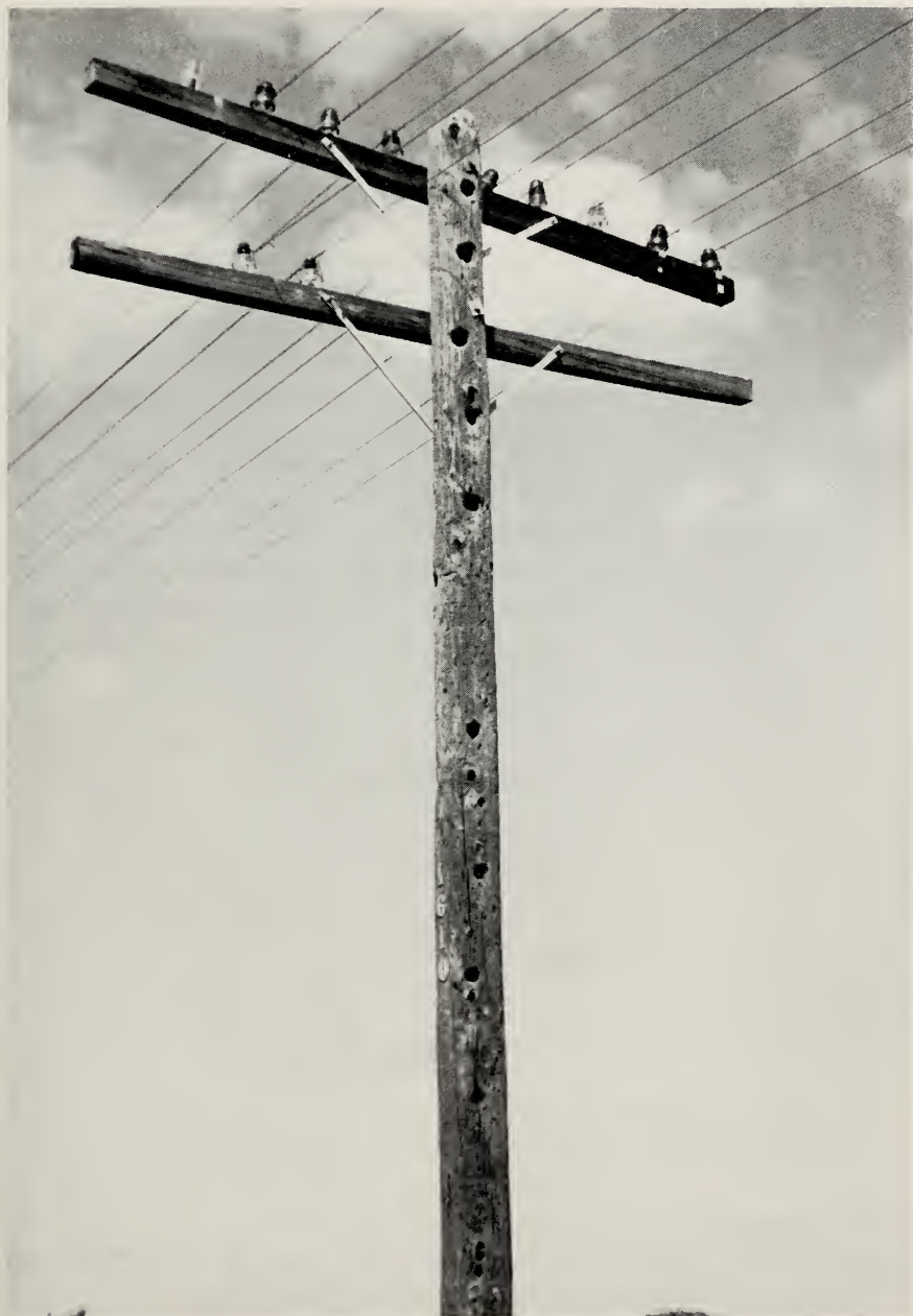
FIG. 2. Distribution of holes on this telephone pole is typical of Ladder-backed's work. Heaviest attack is near the top of pole. A few holes are found on the lower portion and beginning almost from the ground level.
