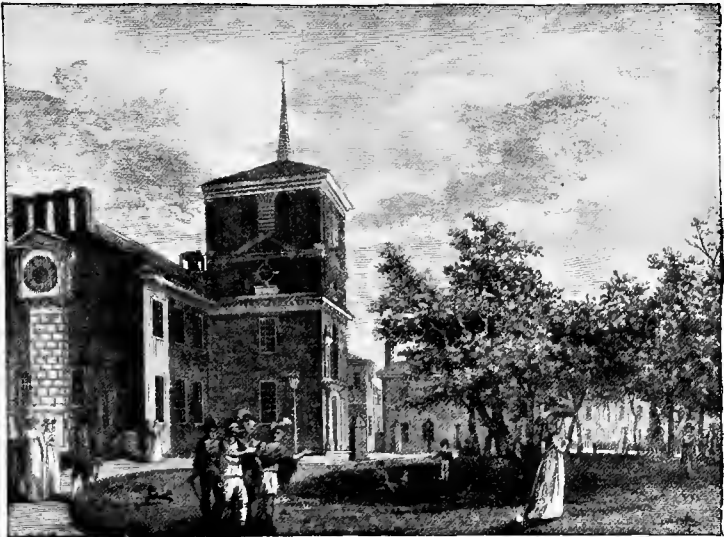
OLD REAR VIEW OF INDEPENDENCE HALL
