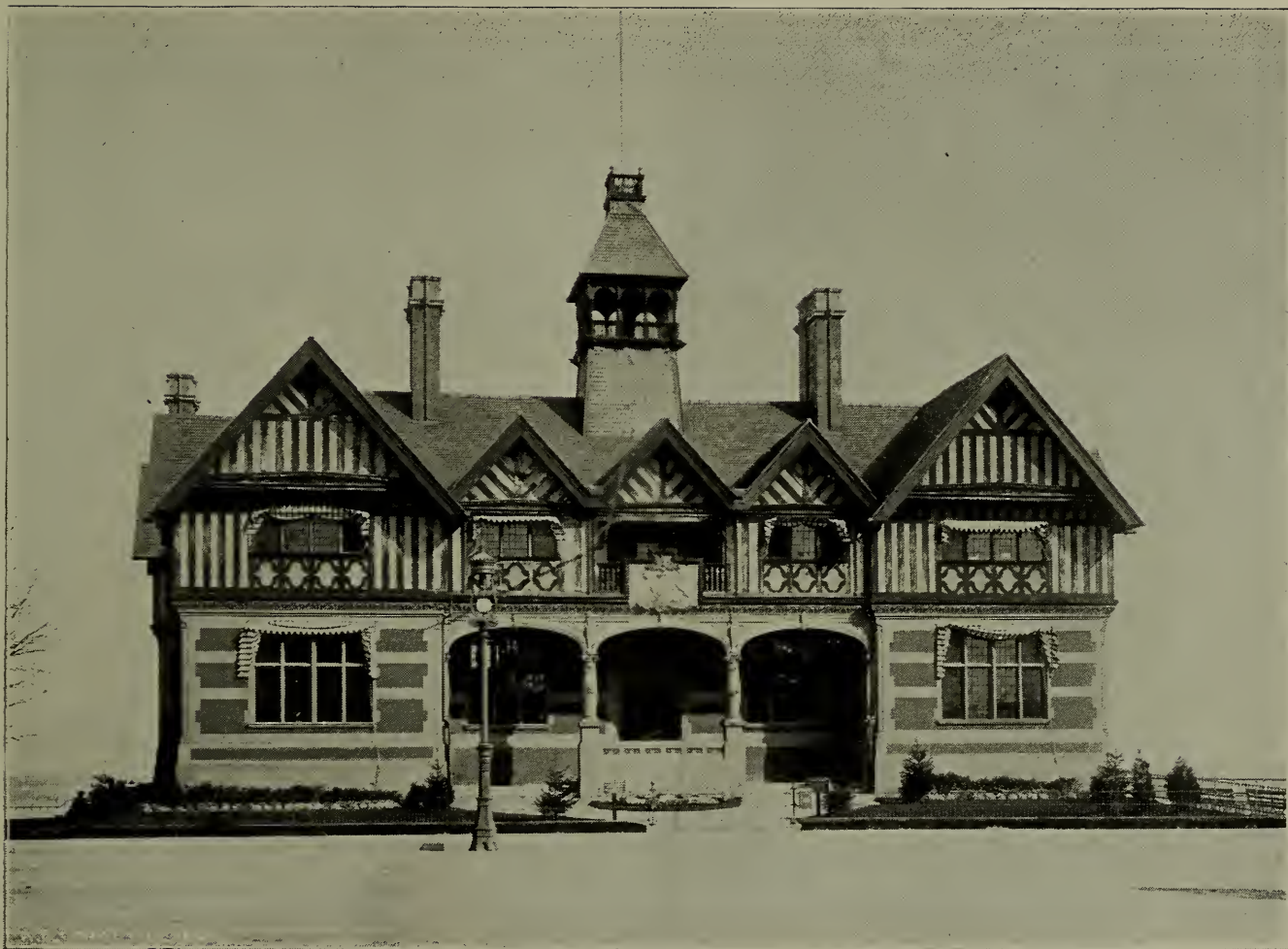
“Victoria House,” as it was called, the headquarters of Great Britain at the Fair, was a picturesque and expensive structure on the lake front, near the famous battle-ship. It was built in the style of the half-timber houses of the time of Henry VIII. It was beautifully decorated and furnished and devoted chiefly to official uses.
