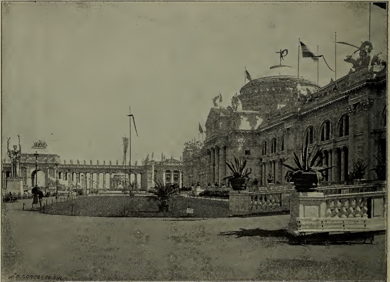
The Agricultural Building never appeared to better advantage than when viewed from the south terrace of the Grand Basin. Here its principal facade with its richness of outlines, wealth of ornamentation, massive Corinthian pillars and statuary of heroic size created an impression which is indelibly impressed on the memory.
