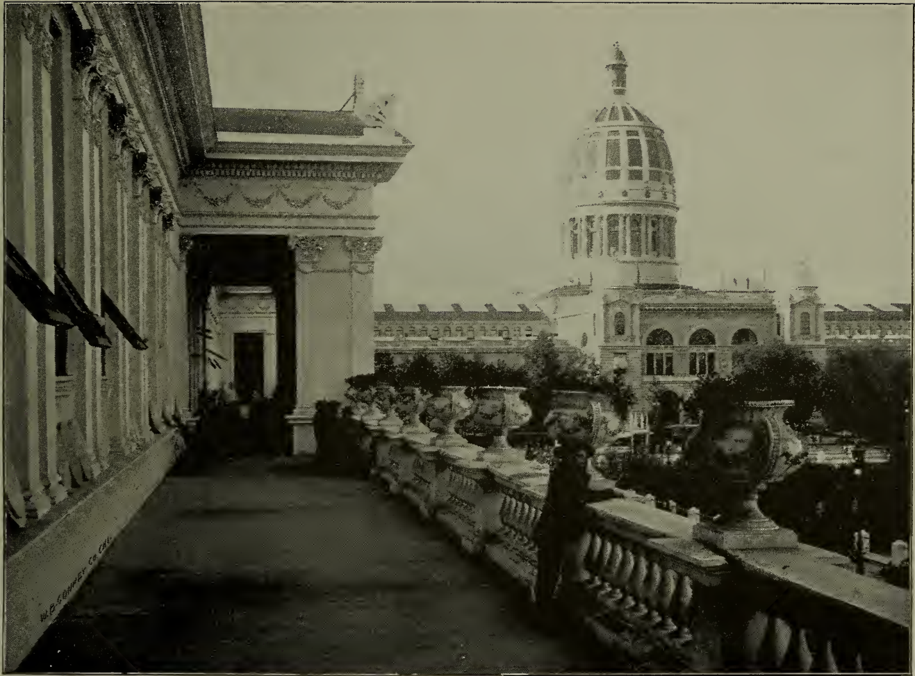
A south view of the Illinois Building from the colonnade of the Woman's Building is produced here with a most artistic effect. The sharpness of outline is softened down by the distance, while the shrubbery in front and the glimpse of the quiet waters of the lagoon give to the whole an Old World appearance
