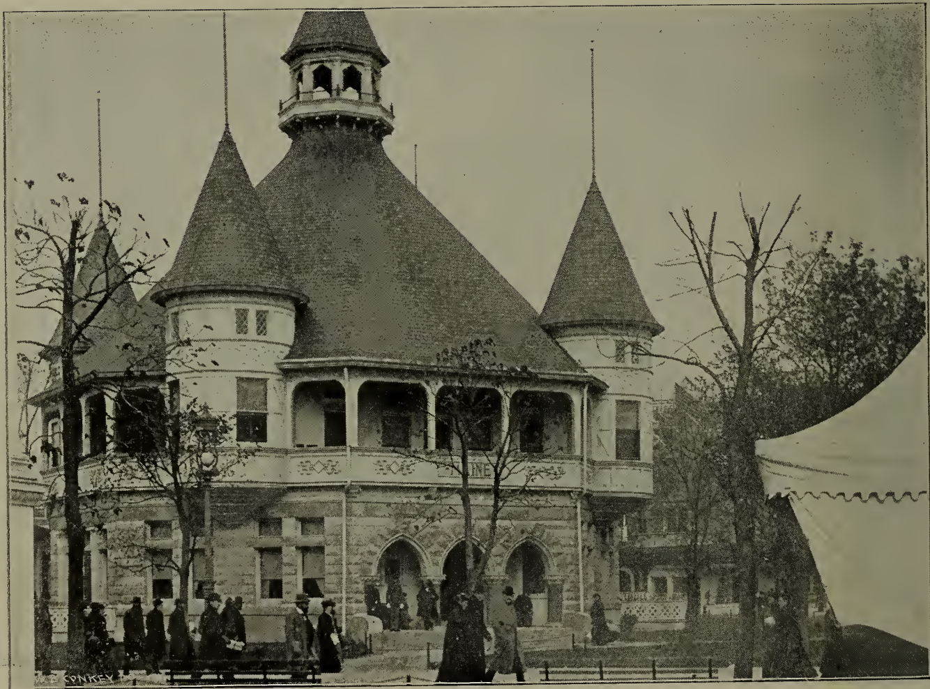
The Maine Building was octagonal in form with an area of sixty-five feet square. The first story was of granite and the exterior of the remainder of the building in wood and staff. The interior finish was handsomely executed in hardwood. The second story projected one foot over the first. The cost was $20,000.
