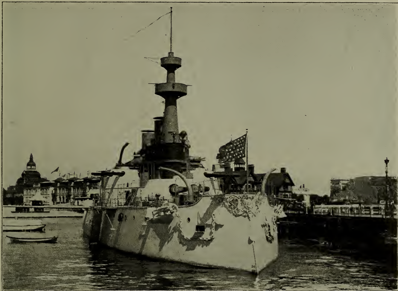
The Battle-Ship Illinois, with its foundation of brick, and its upper works of wood and iron, is said to have been an inspiration of Commodore Meade, of the United States Navy. It was a reproduction in appearance of a genuine battle-ship, and was regularly equipped and manned, forming an instructive object lesson to people living inland.
