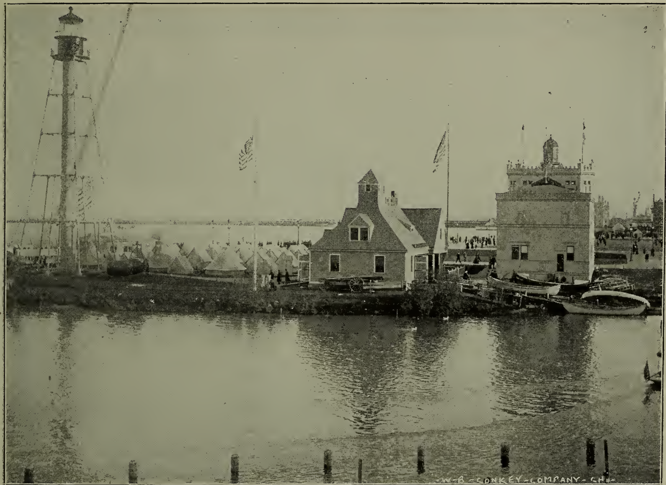
The Naval Observatory, Life Saving Station, Lighthouse Exhibit and Weather Bureau were all grouped near together on the lake front just south of the north inlet. In the illustration the structures devoted to the purposes named appear in the foreground. In the rear is the government encampment. Dimly in the far distance appears the Statue of the Republic.
