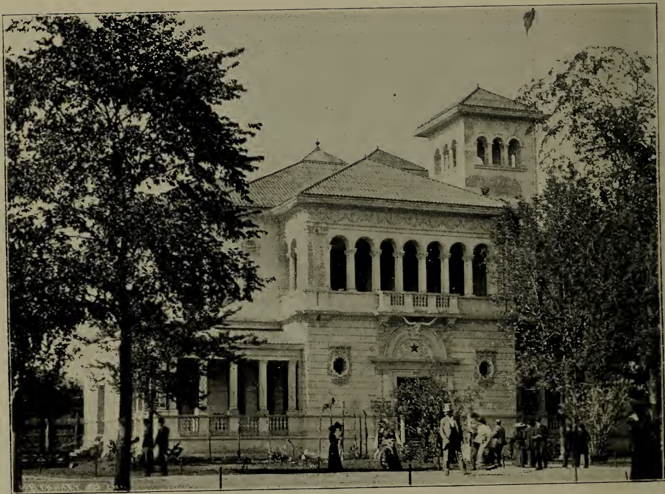
The Texas Building was rather in the Spanish style and stood in the midst of an area beautified by landscape gardening on such a scale as was possible. The assembly room in this building was fifty feet square. It cost $50,000, the money being raised by the Ladies' Auxiliary World's Fair Board of the state.
