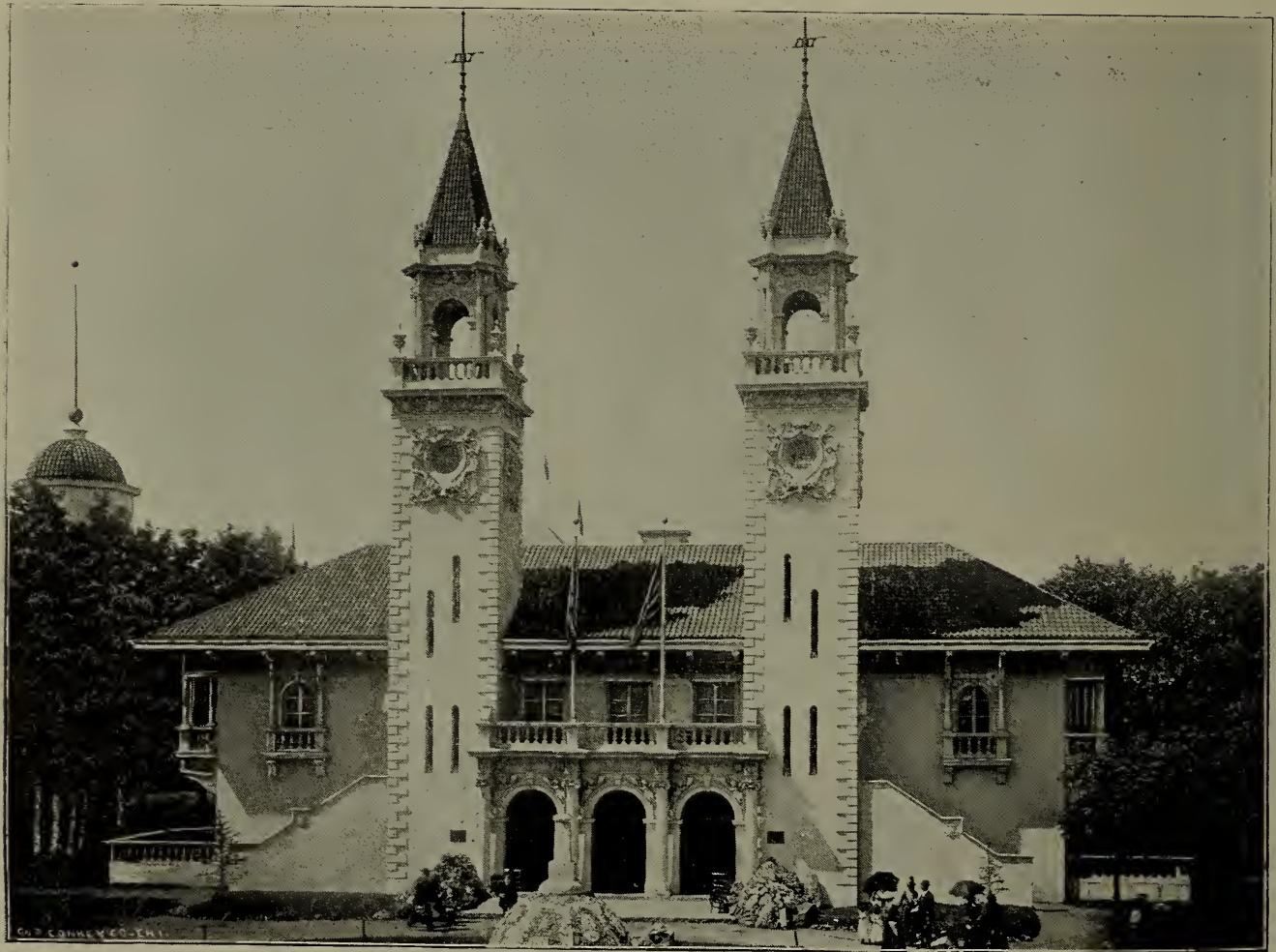
The Colorado Building was in the Spanish Renaissance style of architecture, and was erected at a cost of $35,000. The exterior was of staff of an ivory color. Two slender Spanish towers, ninety-eight feet in height, were noticeable features. The interior was well finished, a splendid onyx mantel being among the decorations. The building was used chiefly as a state headquarters.
