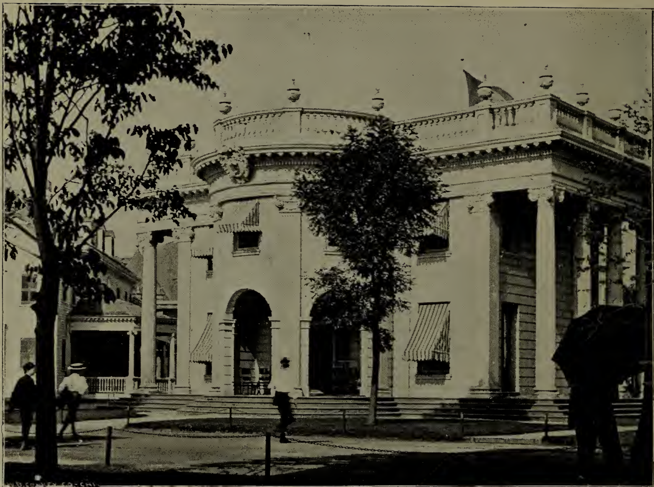
The Rhode Island Building was in the Grecian style, with columnar porticos on four sides. The columns were surmounted by an enriched Ionic entablature, and the building was finished with a roof balustrade. Entrance was had on every side. The structure was devoted, like most of the state buildings, to reception purposes. It cost $10,000.
