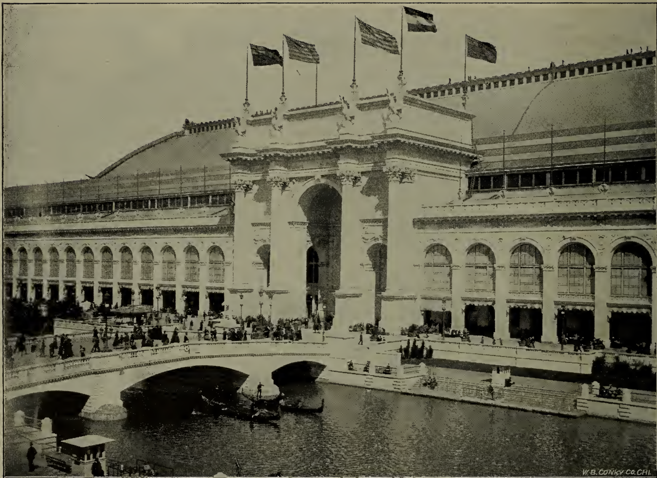
The Manufactures Building had four great entrances, one in the center of each facade. The one here shown is that on the west side and approached by the bridge over the North Canal from Electricity Building. Each entrance was designed after the manner of triumphal arches, the center one being forty feet wide and eighty feet high.
