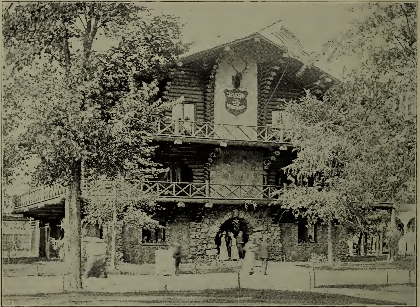
The Idaho Building was in the form of an elaborate Swiss Chalet, though the foundation was of basaltic rock, and the different stories were made of logs stained to give them the appearance of age. Mining and hunting scenes were represented in the interior. The building was sold, to be removed to England after the Fair.
