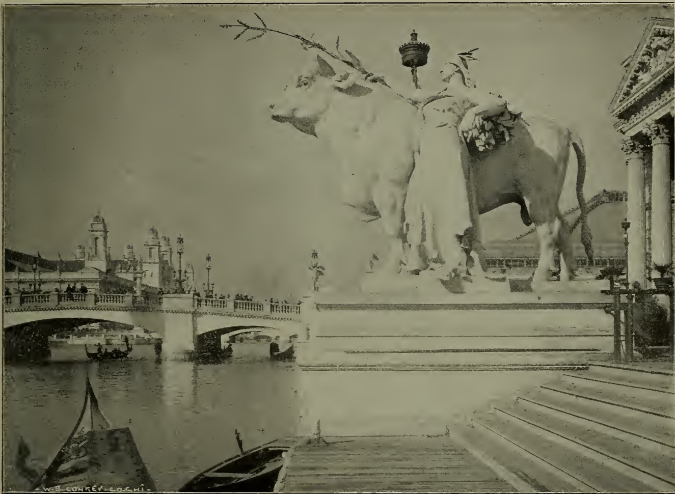
From the west front of the Agriculture Building standing beside one of the statues of Plenty, and looking northwest, the scene was most picturesque in a strictly artificial way. There was nothing of nature to the scene save the water of the canal in front, but the architectural effect was graceful in the extreme.
