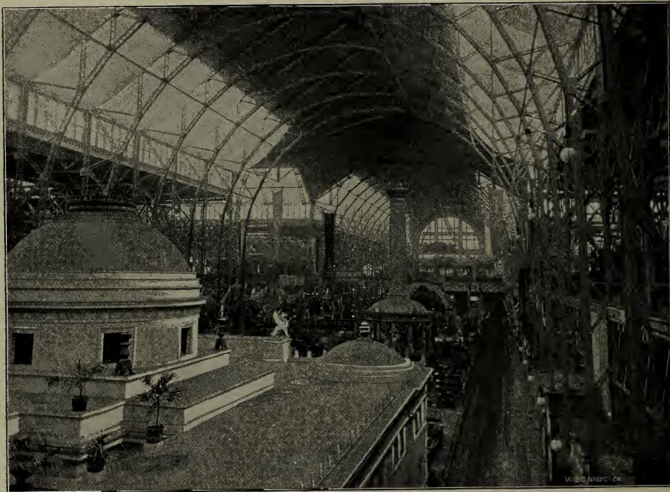
The Interior of the Electricity-Building presented an appearance which would scarcely have been comprehended by visitors to any exposition of the past. Electricity as now applied had not much place a few years ago. In the illustration appears, the telegraph office in the foreground, the column up which colored lights flashed constantly just beyond.
