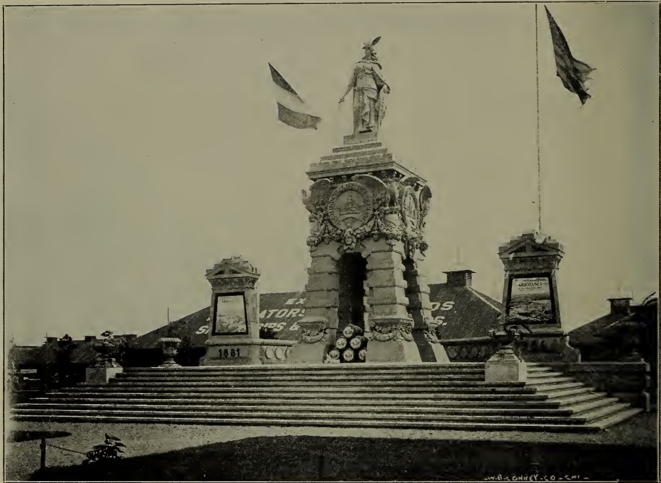
The Statue of Germania, which stood near the stock barns, did not, because of its location, attract the attention it would have done nearer the center of the grounds. The statue had, however, a utilitarian value, since it was cast in cement and served to illustrate to what uses that substance properly constituted may be diverted.
