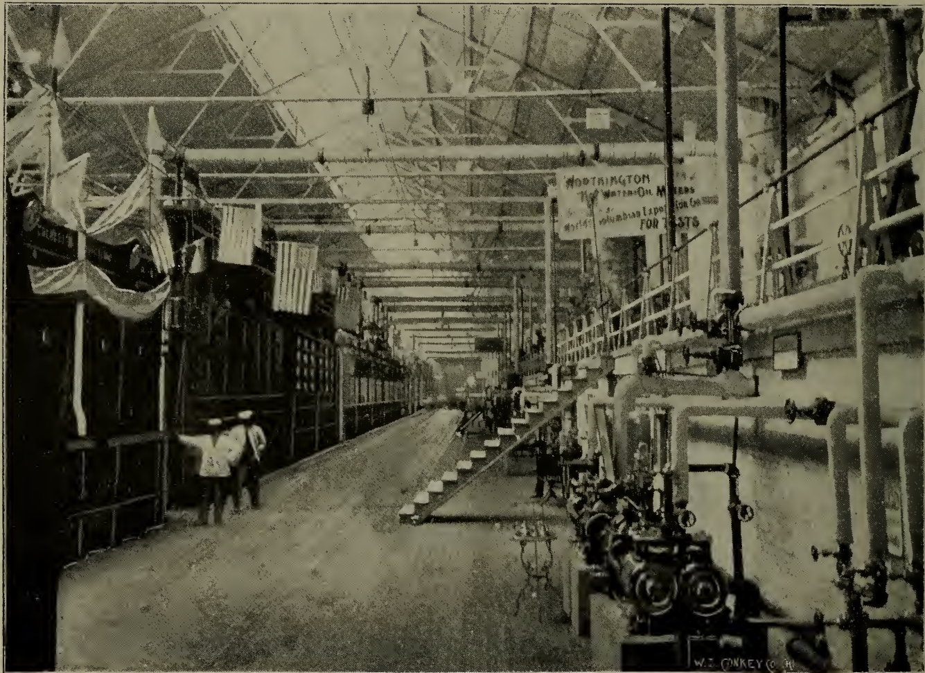
The Boiler Room of Machinery Hall was a sight worth seeing for the student of modern industrial methods. Here was arranged the greatest battery of boilers in the world, the illustration showing its enormous length. No coal was used, the fuel supplied being entirely of kerosene oil. The soul of Watts would have been delighted with the spectacle.
