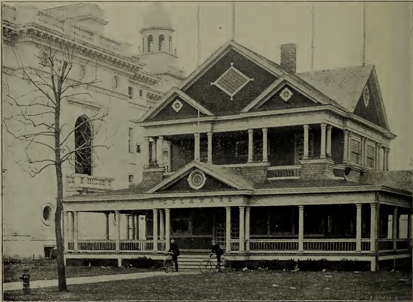
The Delaware Building was constructed of native woods and materials altogether from the state and was erected at a cost of $8,000. It made a picturesque showing, and its interior, one room of which was fitted up in Colonial style, contained many objects of interest, one a figure in clay of the old Swedes church at Wilmington, built one hundred years ago.
