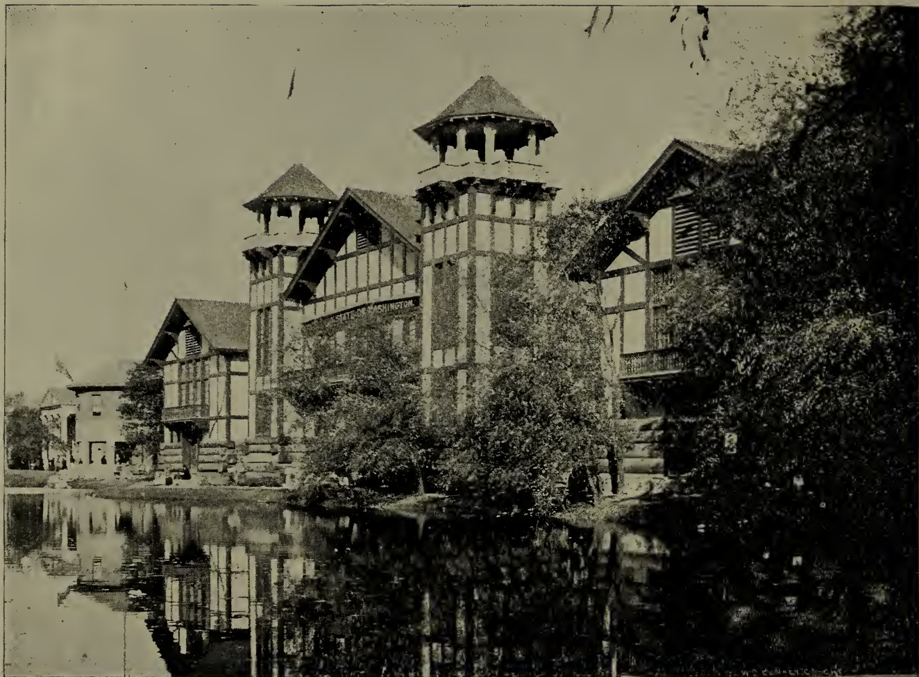
The Washington Building commanded universal attention, constructed, as it largely was, of the gigantic logs of fir brought from the Washington forests. Two base logs were each one hundred and twenty-seven feet long. A monster flagstaff, a single stick, two hundred and eight feet in height, stood in front of the building.
