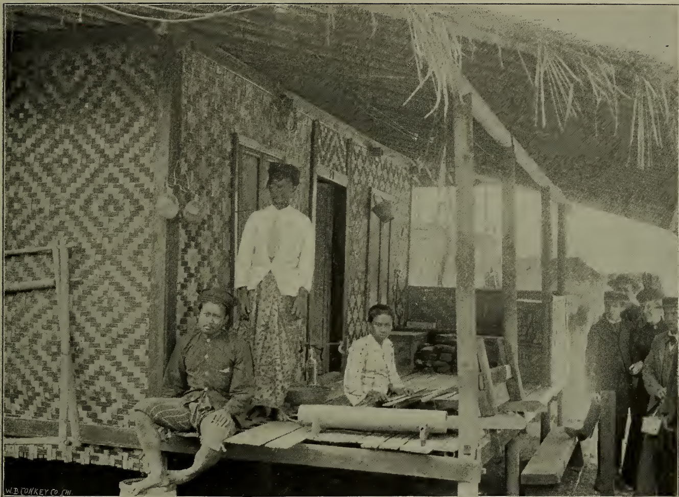
A Javanese House was an interesting object to the visitor. The illustration gives an idea of the style of construction, which must be an excellent one for a warm climate. Bamboo is used almost exclusively, and the house is raised on posts to avoid visits from serpents and similar undesirable guests.
