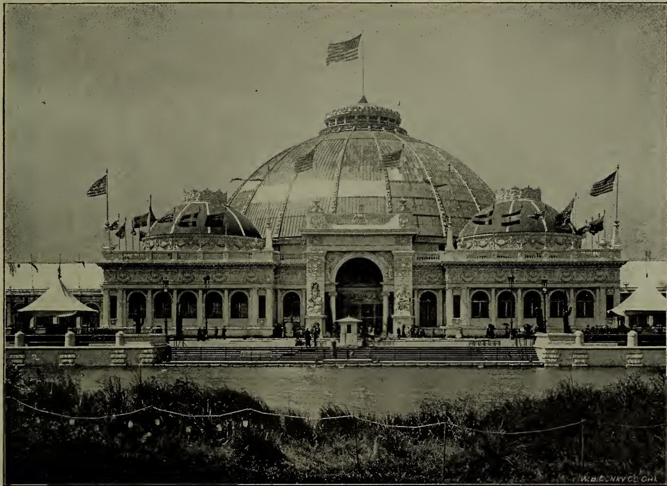
The Horticultural Building, the great storehouse of Flora's treasures at the Exposition, when viewed from the Wooded Island, seemed faultless in its ornate beauty and architectural details. Its style was Venetian Renaissance, the order Ionic. The main entrance was formed by a highly ornamental vestibule, and rising majestically above it was the crystal dome one hundred and thirteen feet high and one hundred and eighty-seven feet in diameter.
