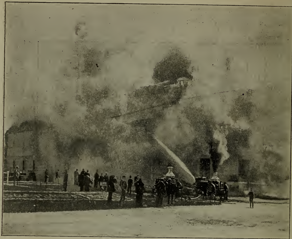
The struggle with the flames on the occasion of the Cold Storage Warehouse fire in the Fair grounds was a helpless one. Of the men cut off from escape, sixteen were lost and several others were more or less seriously injured. At least fifty thousand horrified spectators were witnesses of the appalling scene.
