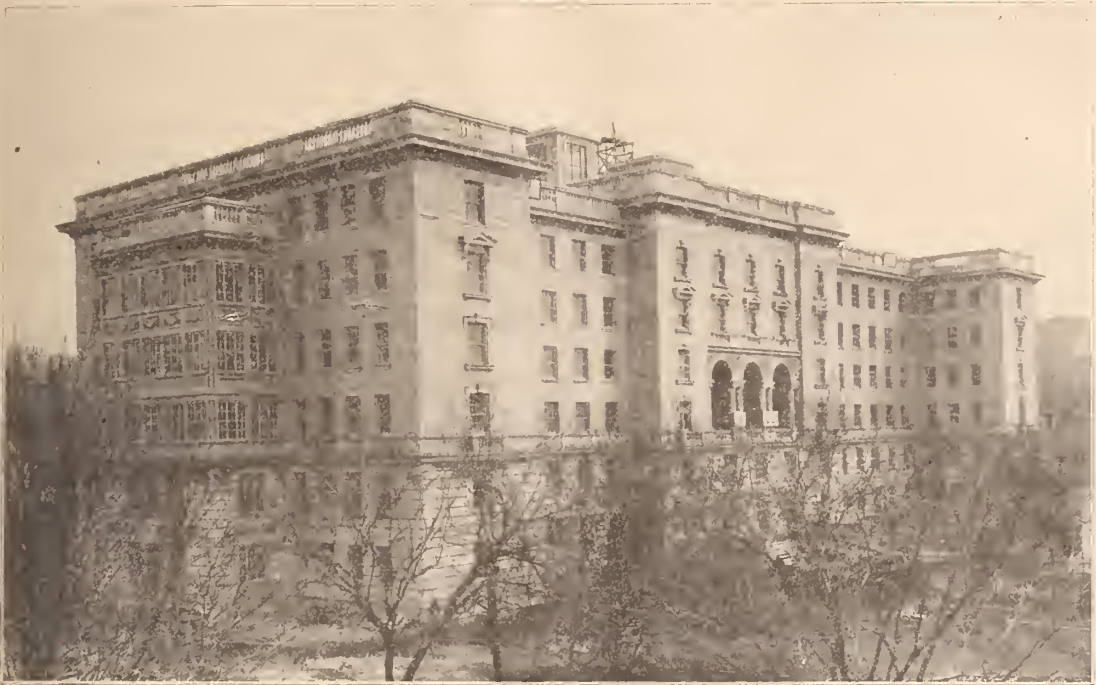
STATE OF WISCONSIN GENERAL HOSPITAL, UNIVERSITY OF WISCONSIN, MADISON
