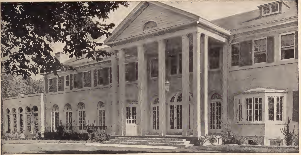
COLONIAL HALL—One of Eight Units in "cottage plan"
