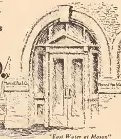
"East Water at Mason"
