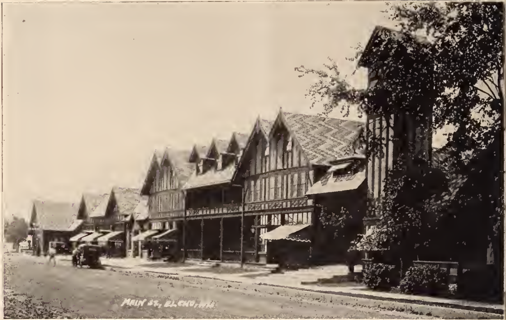
The village of Elcho, Langlade county, Wisconsin, was composed, not many years ago, of squalid, old and unsightly buildings. Charles W. Fish recently rebuilt the town into the beautiful Nuremberg village shown here.
