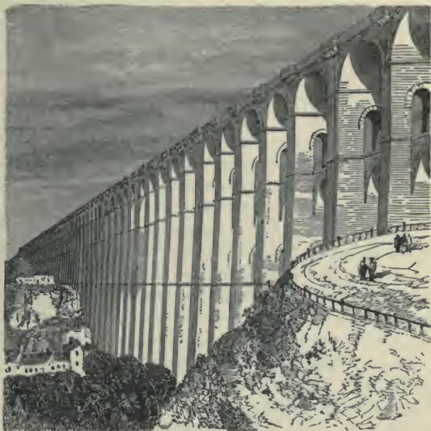
Viaduct of Chaumont.
