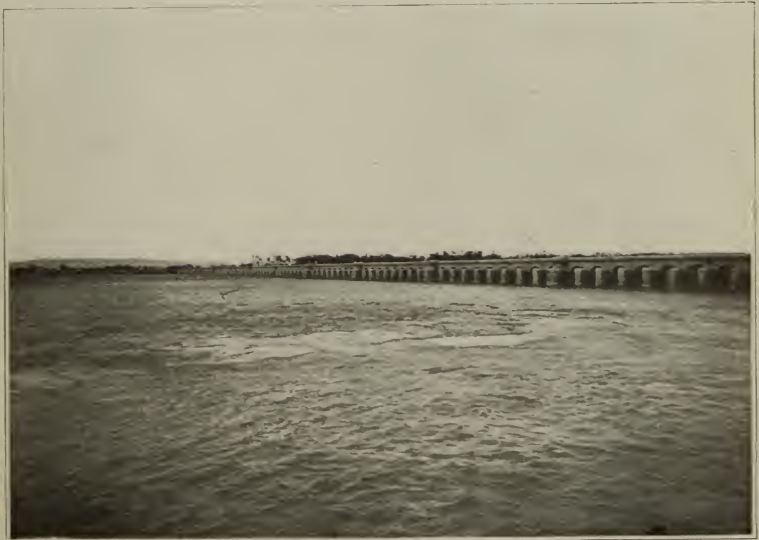
FIG. 2.—THE ASSIUT BARRAGE ACROSS THE NILE.
