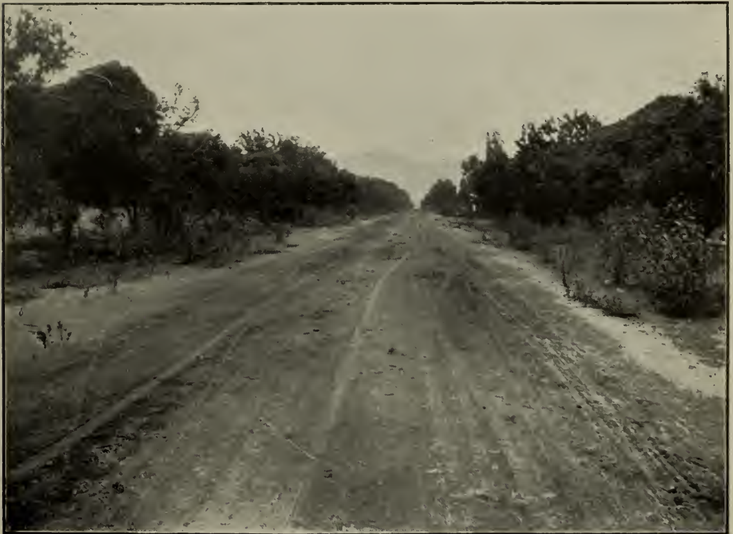
FIG. 2.—SAME ROAD SHOWN IN FIG. 1; AFTER OILING HAS HARD, SMOOTH CRUST.
