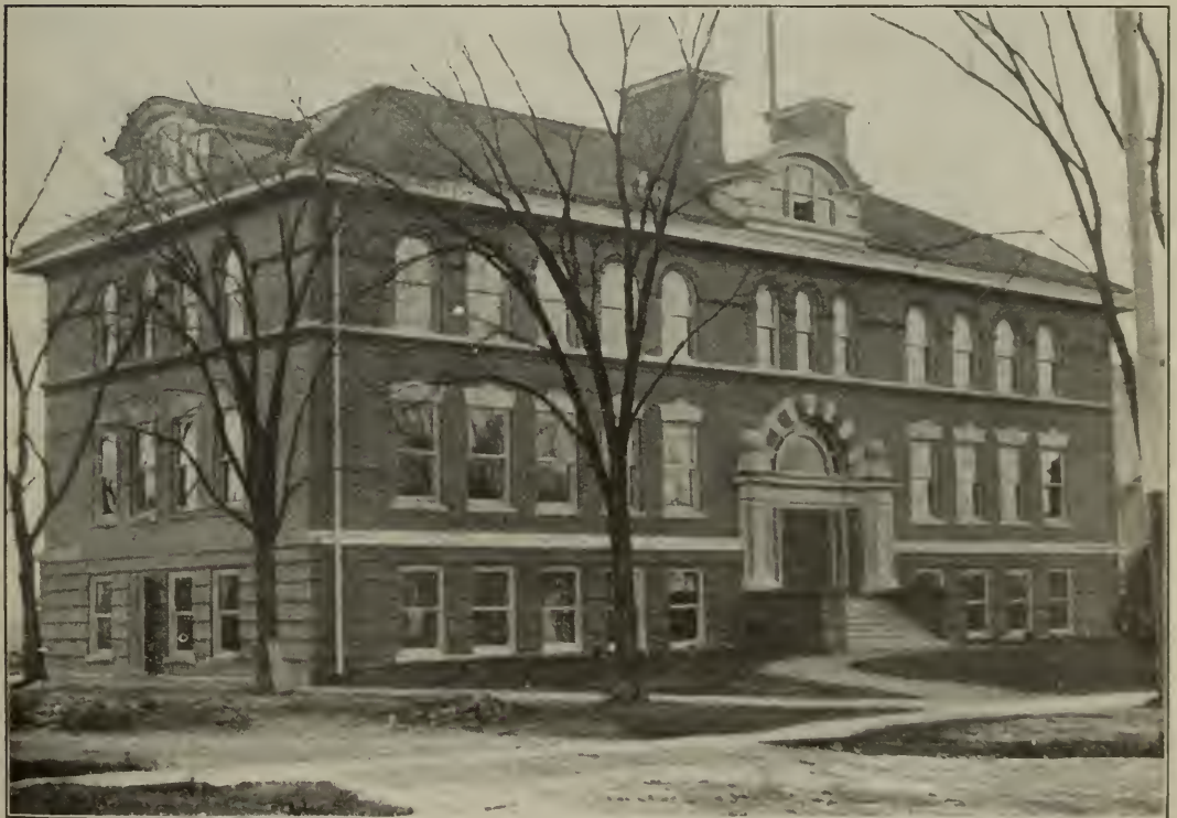
FIG. 2.—MAIN BUILDING OF THE DUNN COUNTY SCHOOL OF AGRICULTURE AND DOMESTIC SCIENCE, MENOMONIE, WIS.
