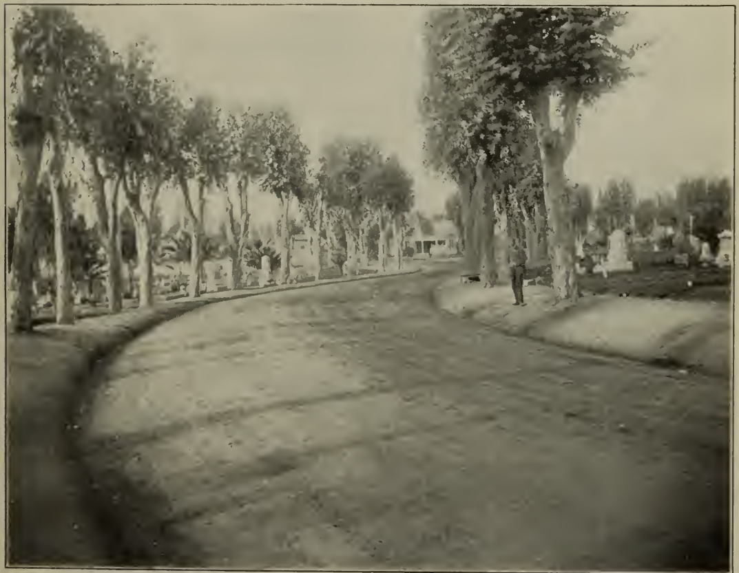
FIG. 2.—ROAD IN EVERGREEN CEMETERY, LOS ANGELES, CAL., OIL SURFACE NEWLY FINISHED.
