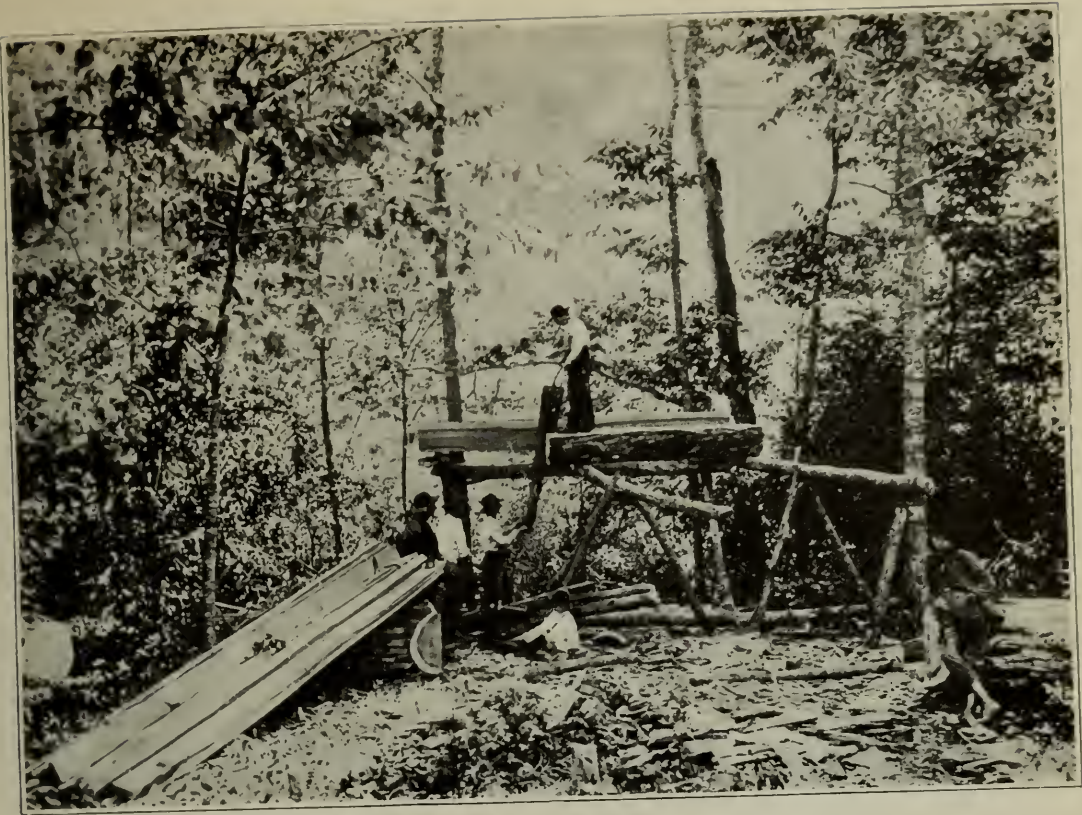
FIG. 1.—WHIP SAWING IN THE KENTUCKY MOUNTAINS.
