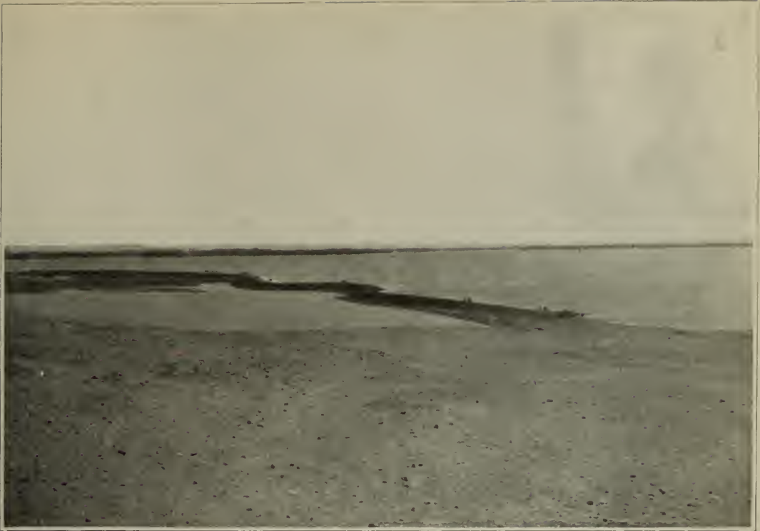
FIG. 1.—BASIN IRRIGATION IN EGYPT. [The bank between the two basins is used as a road.]
