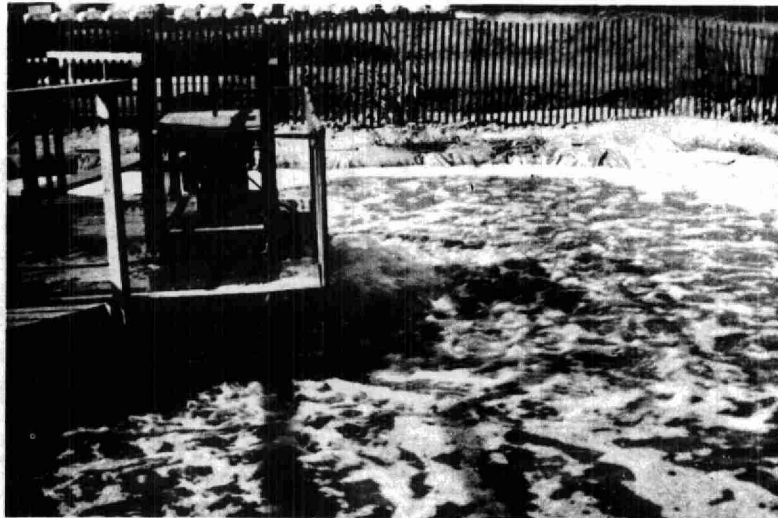
Figure 14 Operation of lagoon #3 during tomato pack.
